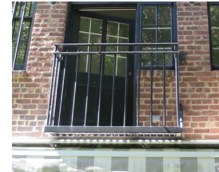
EXISTING CONDITIONS AT PARLOR FLOOR (NEW RAILING TO MATCH)
