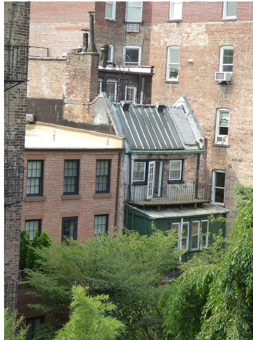
3. VIEW LOOKING SOUTH WEST FROM ROOF - ENLARGED
