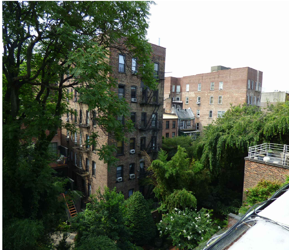
2. VIEW LOOKING SOUTH WEST FROM ROOF
