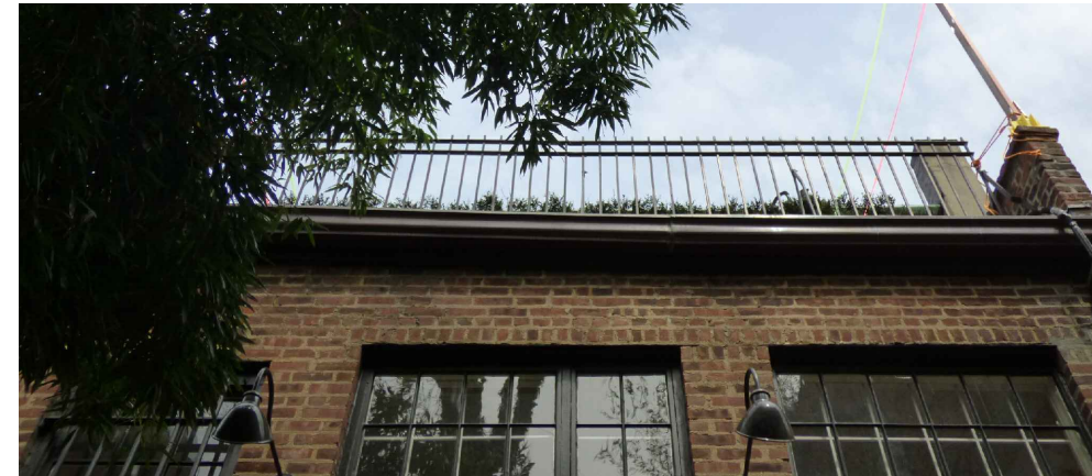
EXISTING REAR TERRACE RAILING
