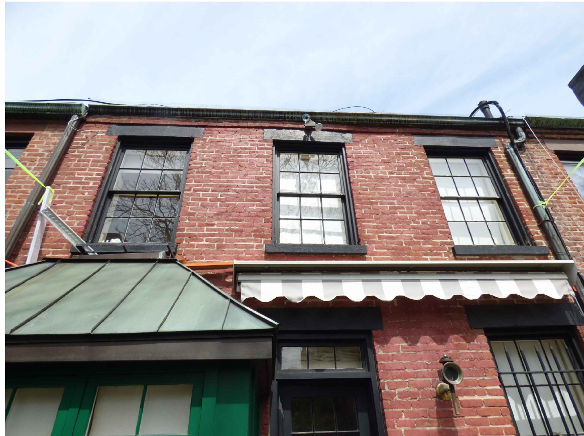
EXISTING 4TH FLOOR REAR WINDOWS
