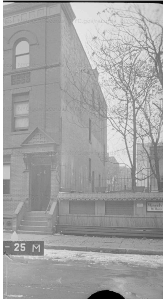
NYC TAX PHOTOGRAPHS, CA. 1940 VIEW CORRIDOR TO REAR FROM WAVERLY PLACE
