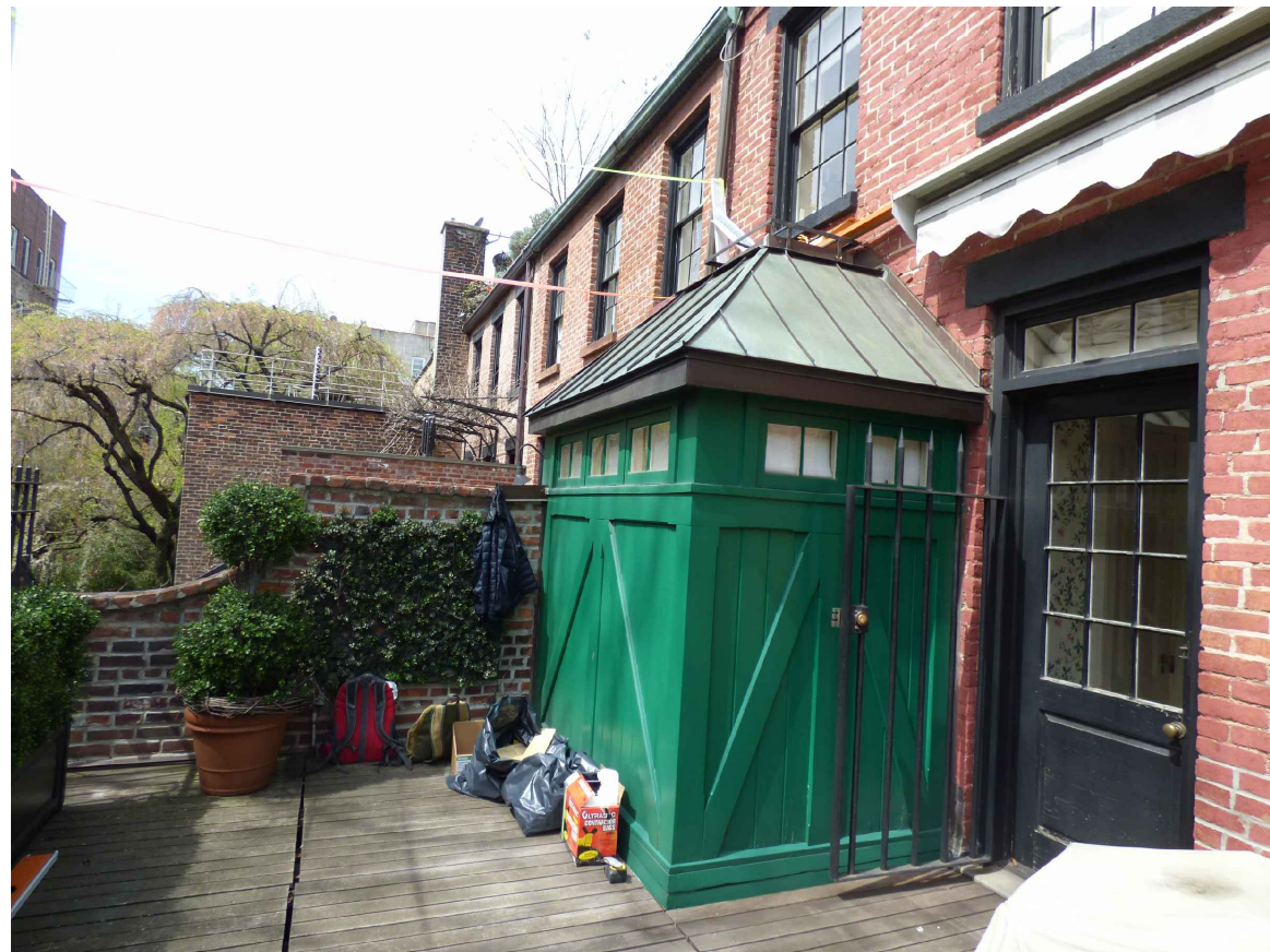
EXISTING TERRACE VIEW LOOKING WEST
