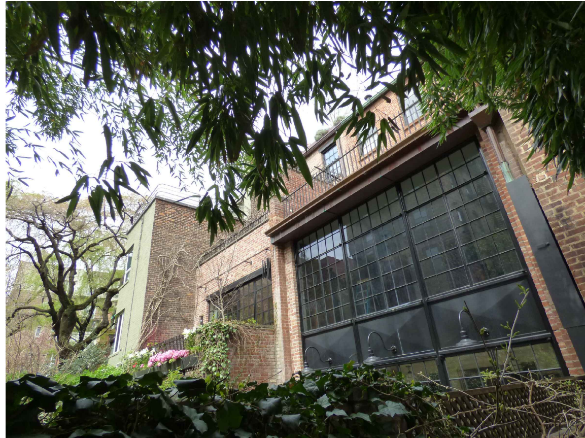
1. VIEW OF NEIGHBORING BUILDING TO THE WEST (24 BANK STREET)
