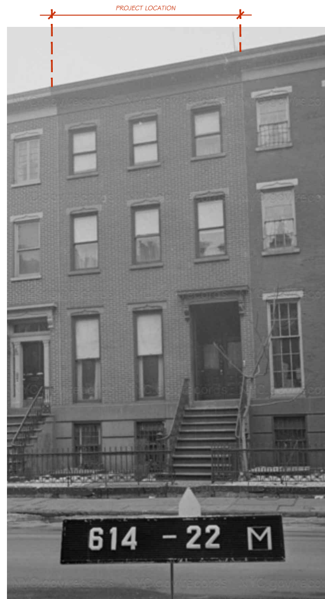
FRONT FACADE - CA 1940
