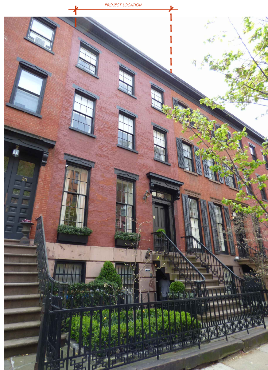
EXISTING FRONT FACADE
