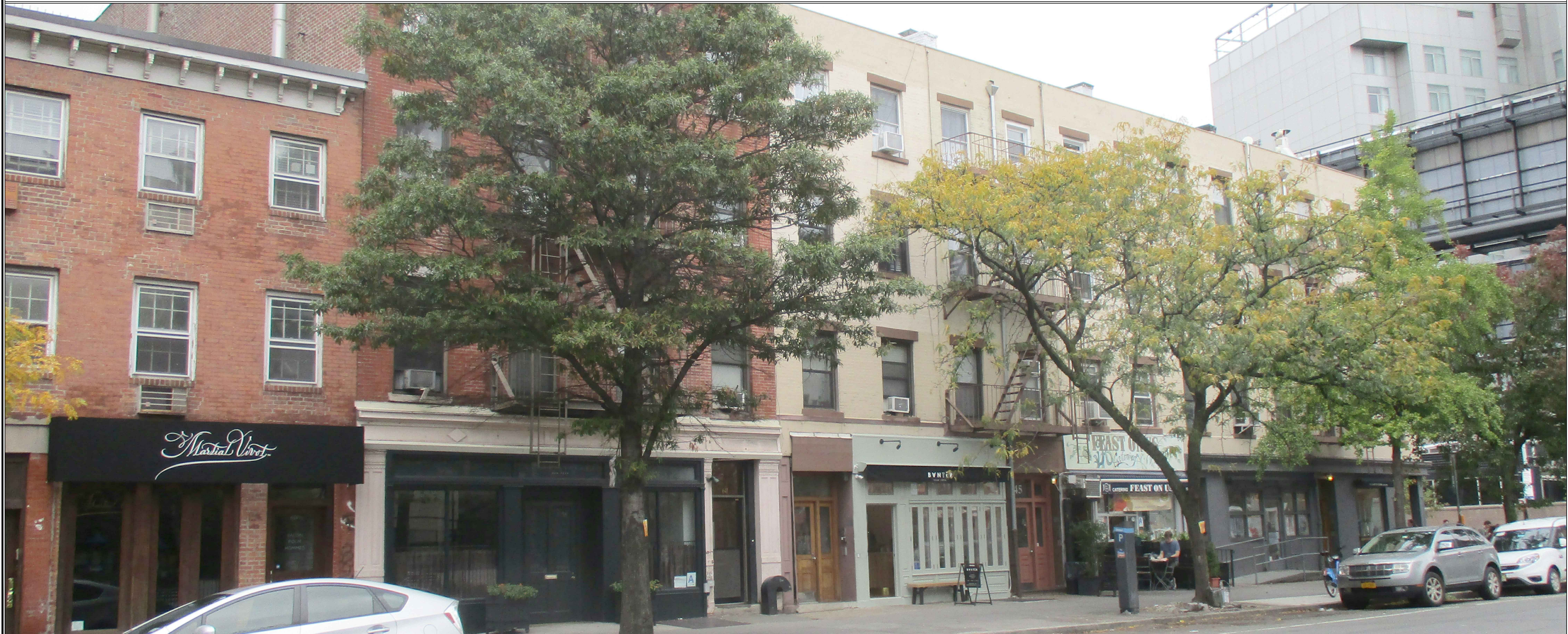
EXISTING CONDITIONS PHOTO (NOV 2019)
