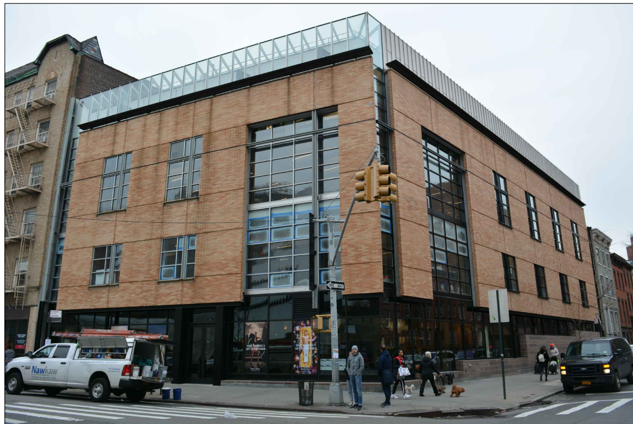
WORK APPROVED UNDER LPC COFA 19-38470 IS IN PROGRESS
