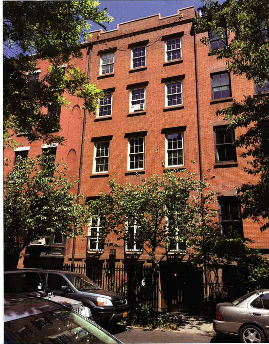
04 CURRENT CONDITION PHOTO, 2016 LC-01 NTS
