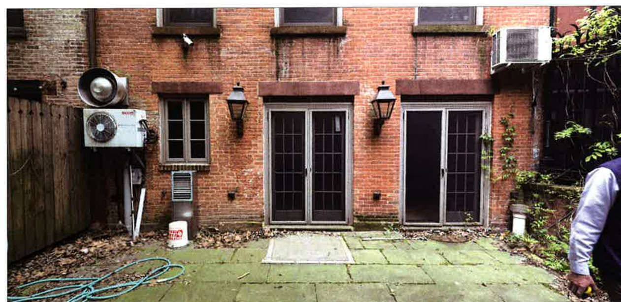
01 EXISTING REAR ELEVATION - VIEW OF BASEMENT FLOOR AT REAR GARDEN LC-14
