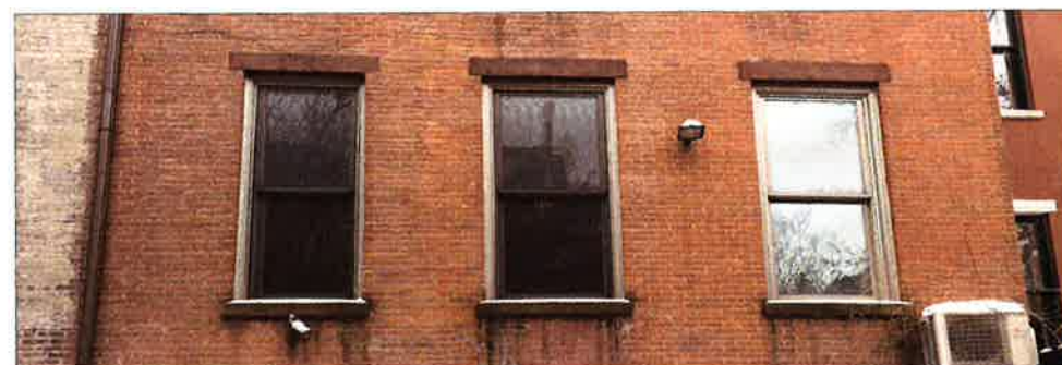
02 EXISTING REAR ELEVATION - VIEW OF 1ST FLOOR WINDOWS LC-14
