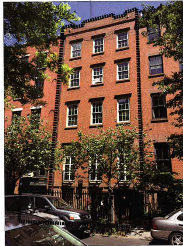
03 LC-02 VIEW FROM ACROSS THE STREET LOOKING NORTHWEST
