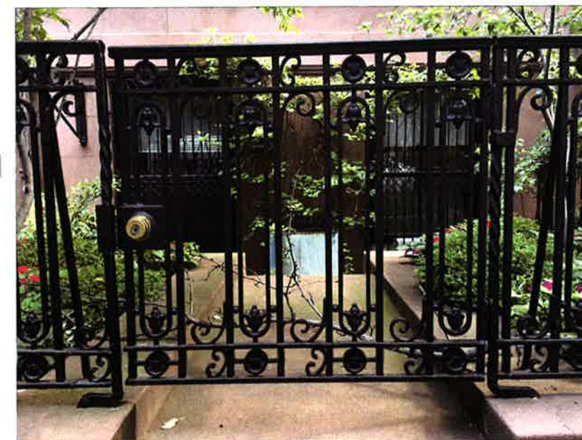
05 PHOTO OF EXISTING AREAWAY FENCE AT 19 W 10TH STREET LC-08
