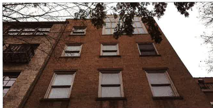
03 EXISTING REAR ELEVATION - VIEW OF 2ND THROUGH 4TH FLOOR WINDOWS LC-14
