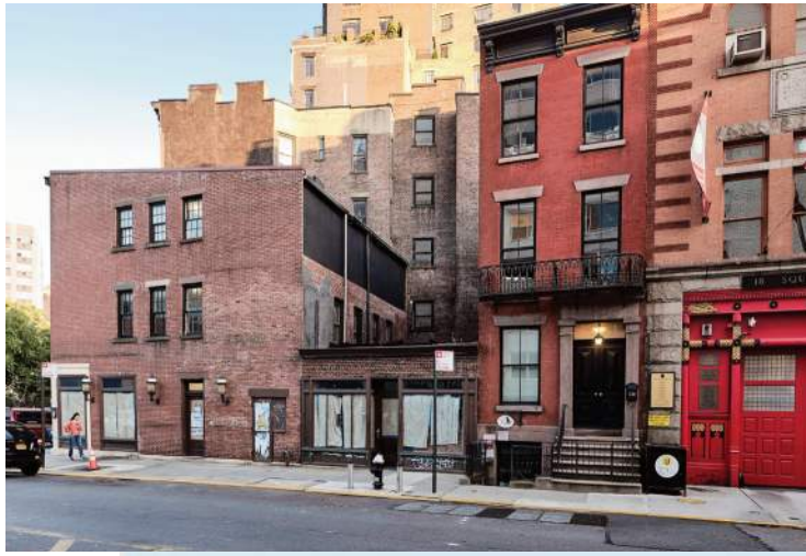
EXISTING WEST 10TH STREET FACADE (2019)
