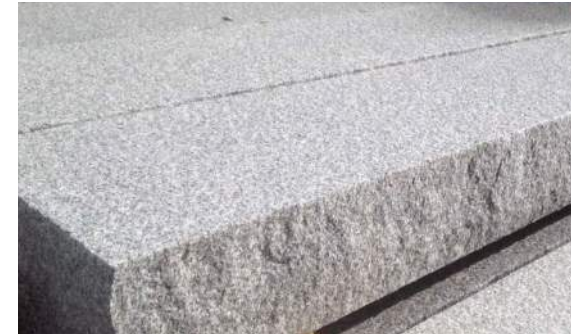
EXISTING GRANITE PIERS TO BE RESTORED TO ORIGINAL COLOR
