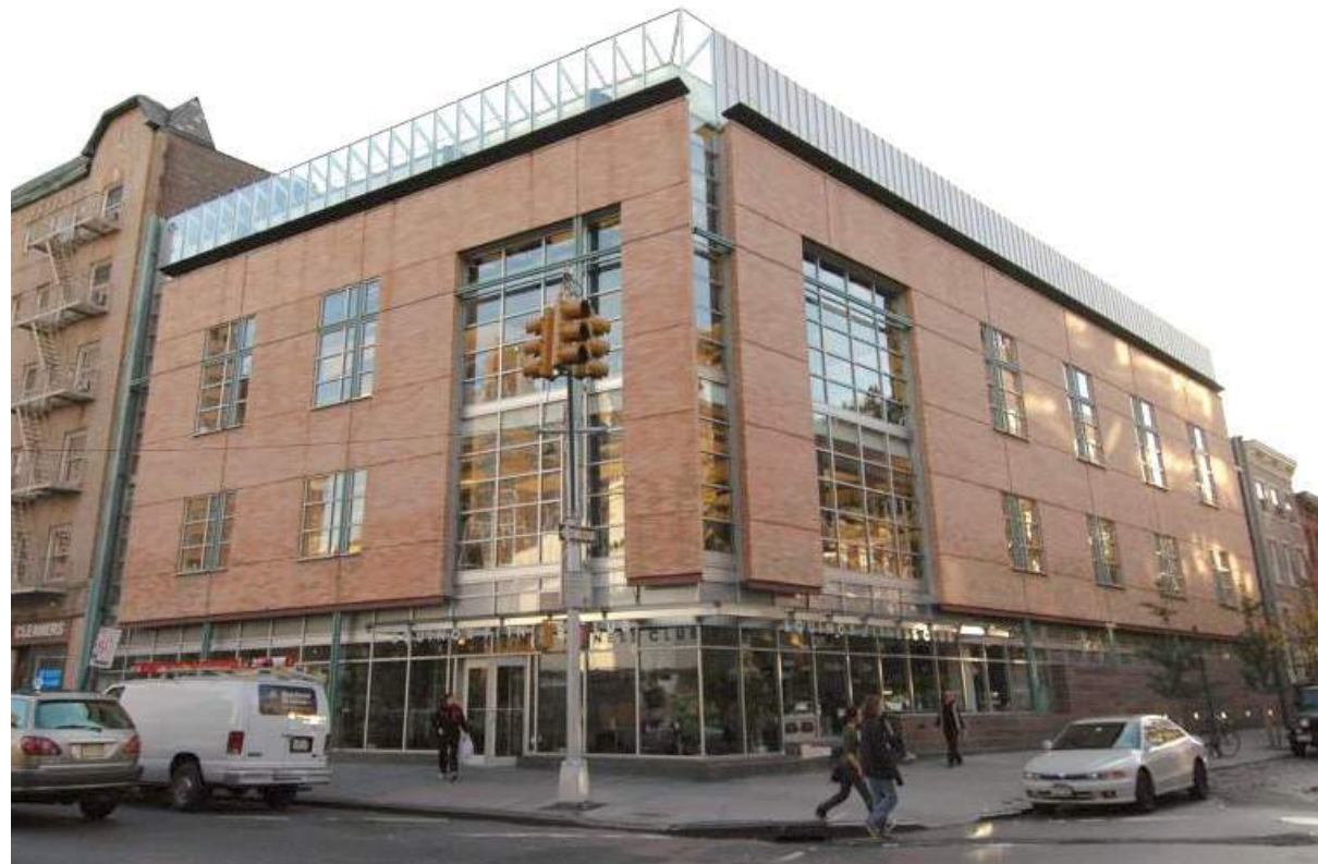
97 GREENWICH AVENUE, LPC APPROVAL, 2000, PLATT BYARD DOVELL ARCHITECTS
