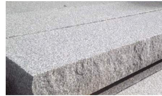
EXISTING GRANITE PIERS TO BE RESTORED TO ORIGINAL COLOR
