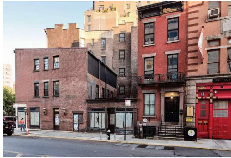
EXISTING WEST 10TH STREET FACADE (2019)
