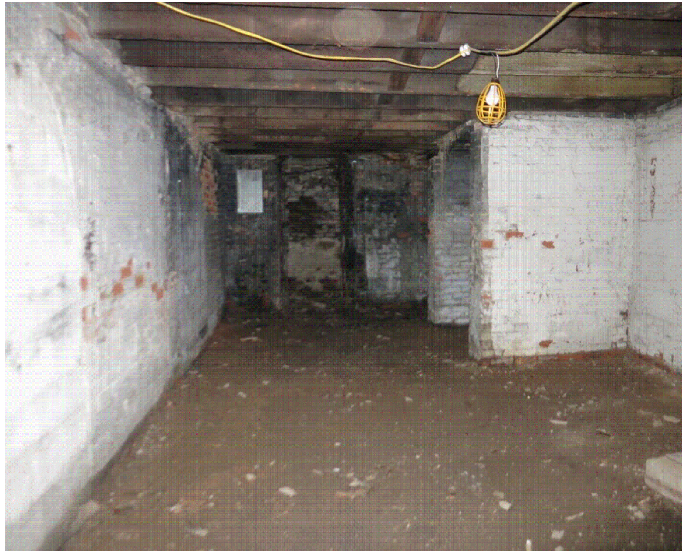
4. EXISTING BASEMENT BACK WALL
