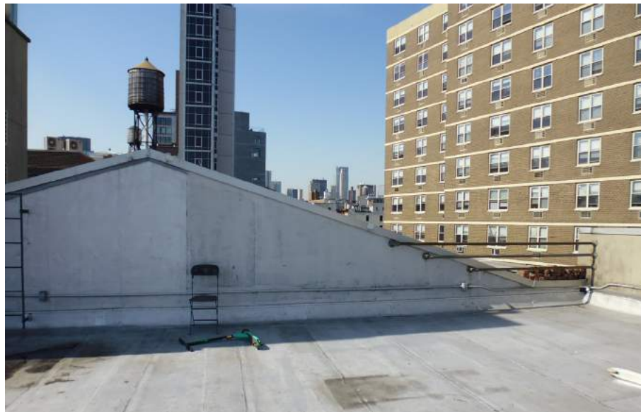
Existing gabled parapet and ladders to remain
