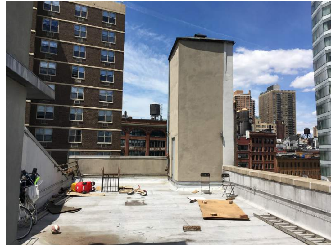
Existing bulkhead tower view
