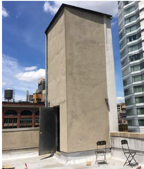
Existing bulkhead tower view from terrace
