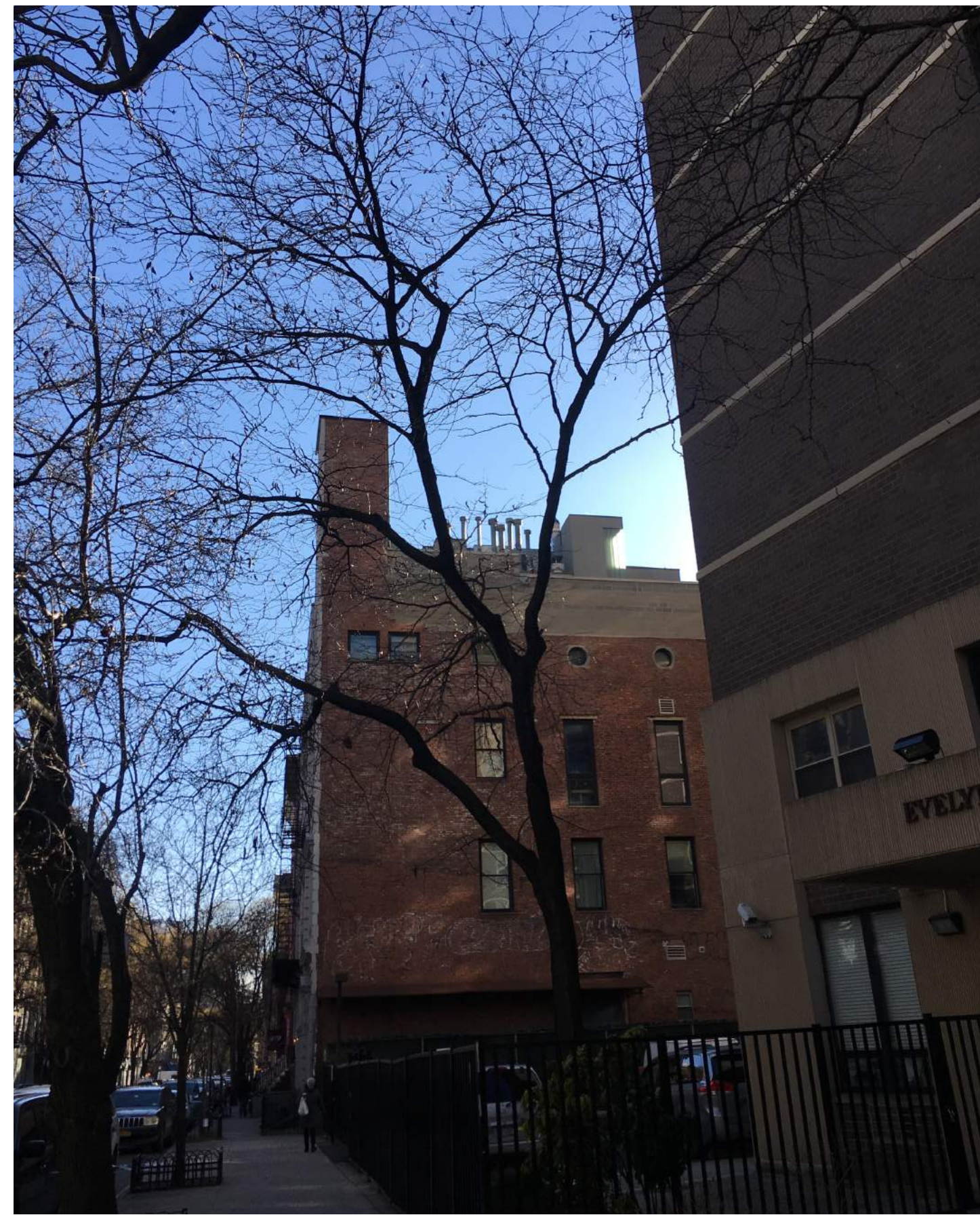
SECONDARY FACADE FROM EAST 5TH STREET
