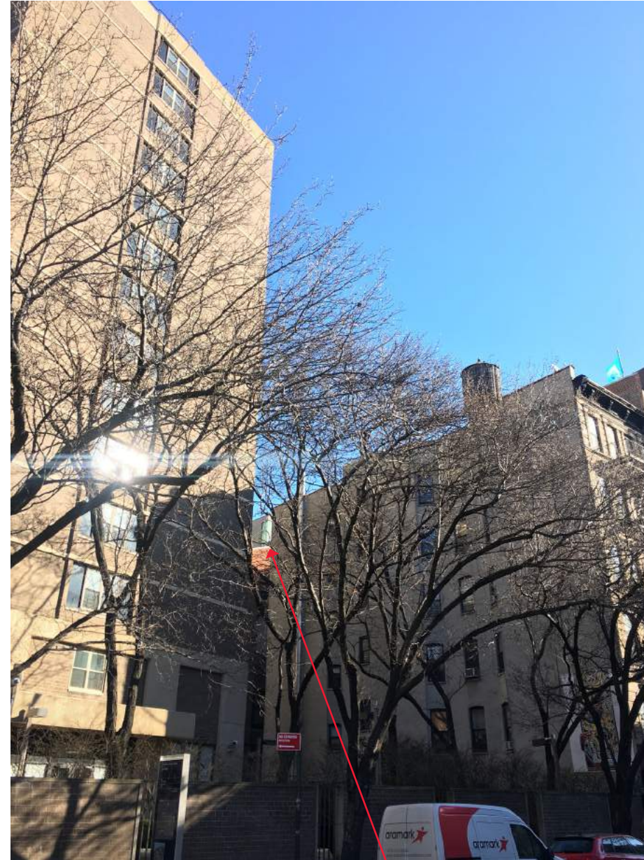
14 210 EAST 5TH STREET- EXISTING STAIR VISIBLE BETWEEN BUILDINGS
