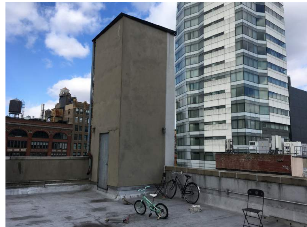
Existing bulkhead tower view
