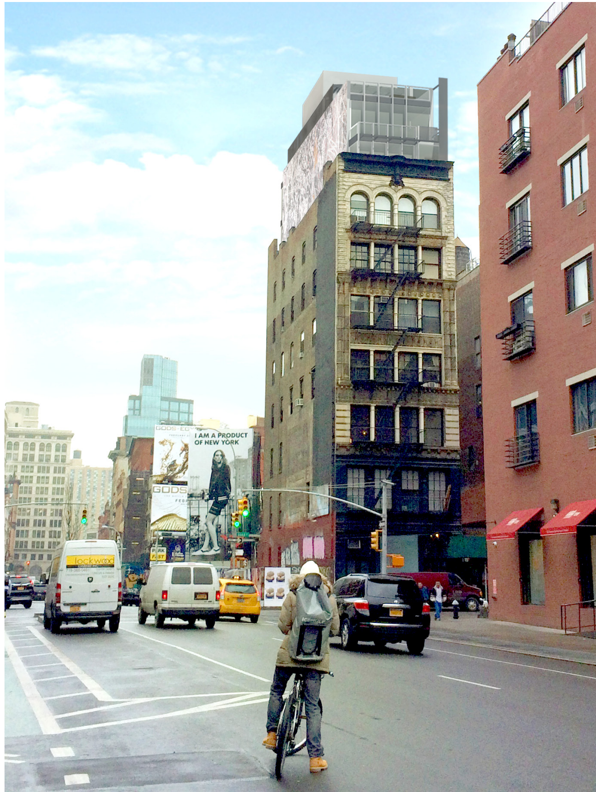
VIEW FROM SOUTH, LAFAYETTE ST. AND BOND ST. INTERSECTION OF APPROVED DESIGN
