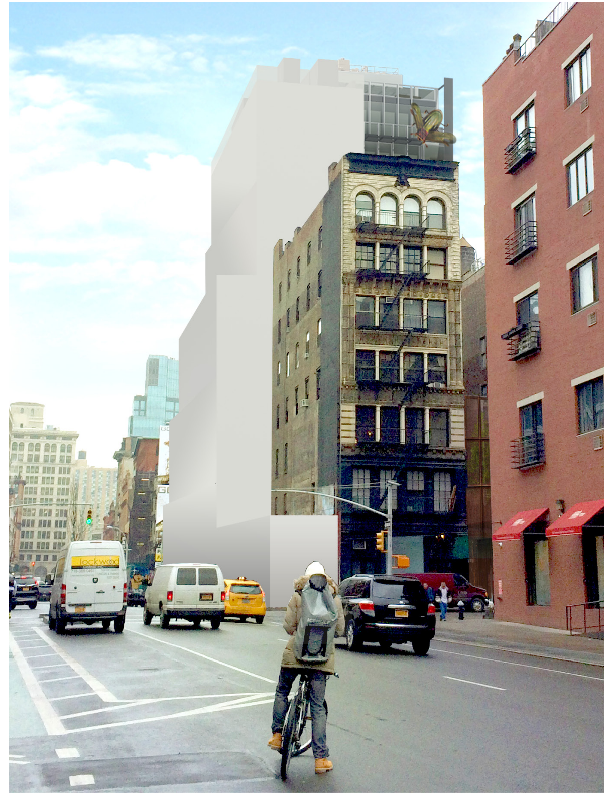
VIEW FROM SOUTH, LAFAYETTE ST. AND BOND ST. INTERSECTION SHOWING PROPOSED ARTWORK (WITH PROPOSED MASSING OF 355 LAFAYETTE)
