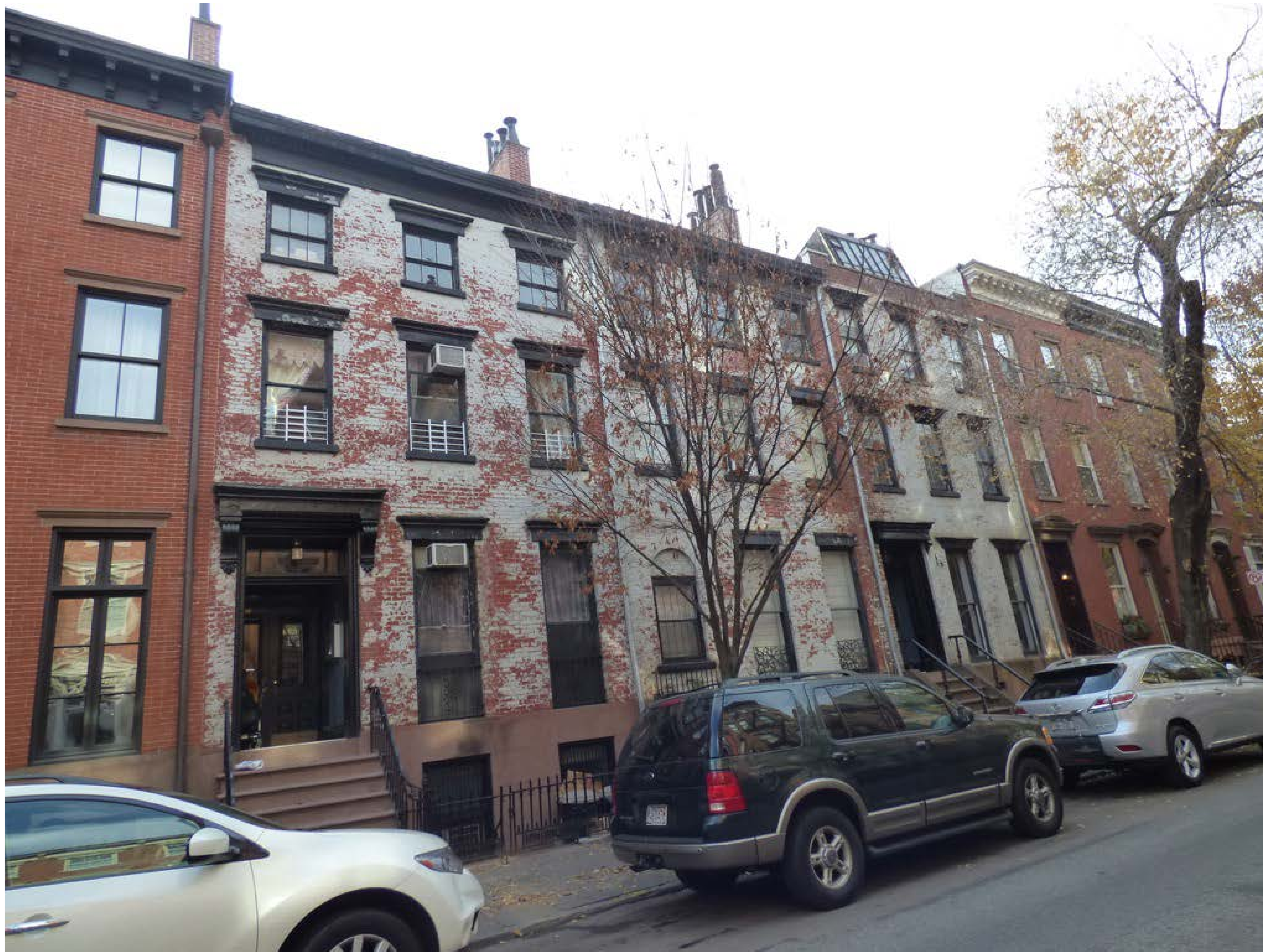
242-246 WEST 11TH STREET BUILT 1842
