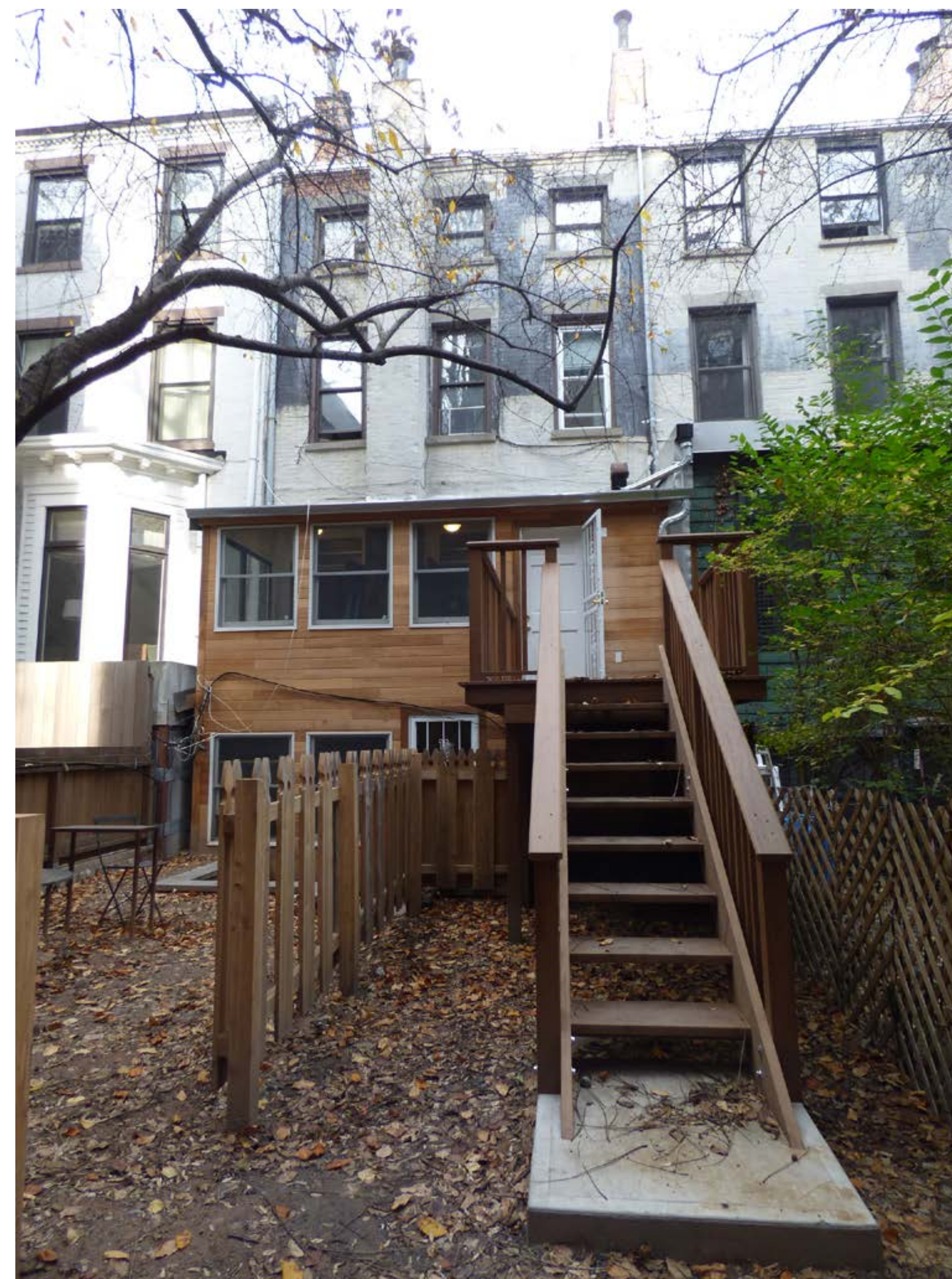
246 WEST 11TH STREET - REAR ELEVATION
