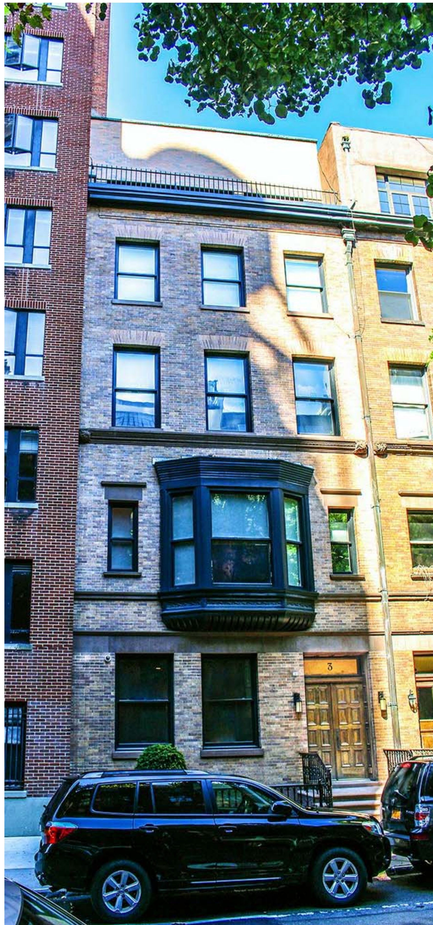
1 FRONT FACADE EXISTING 1" = 50'-0"
