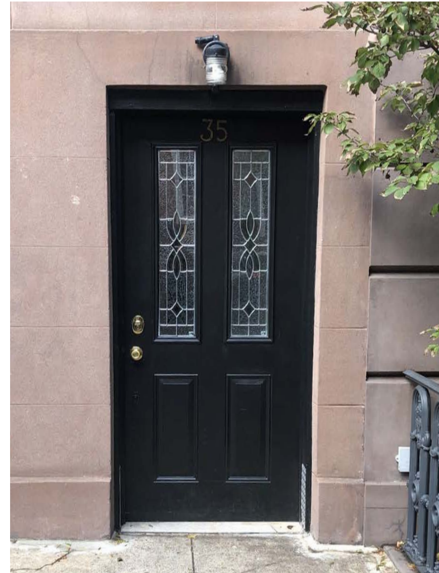
35 CHARLES STREET MAIN ENTRANCE
