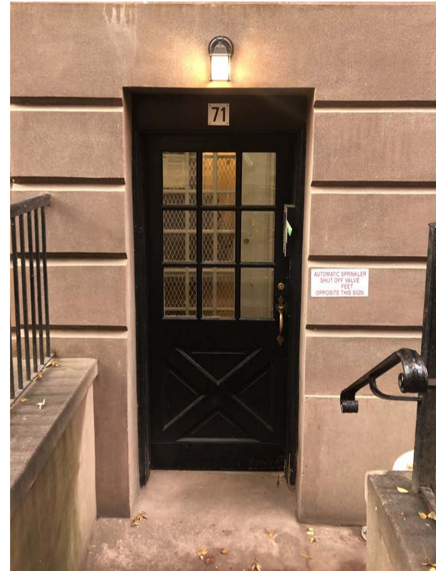
71 CHARLES STREET MAIN ENTRANCE
