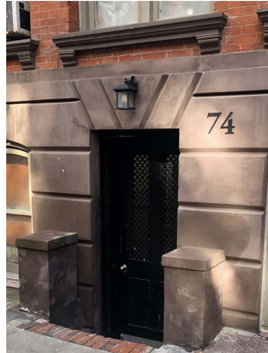
74 CHARLES STREET MAIN ENTRANCE
