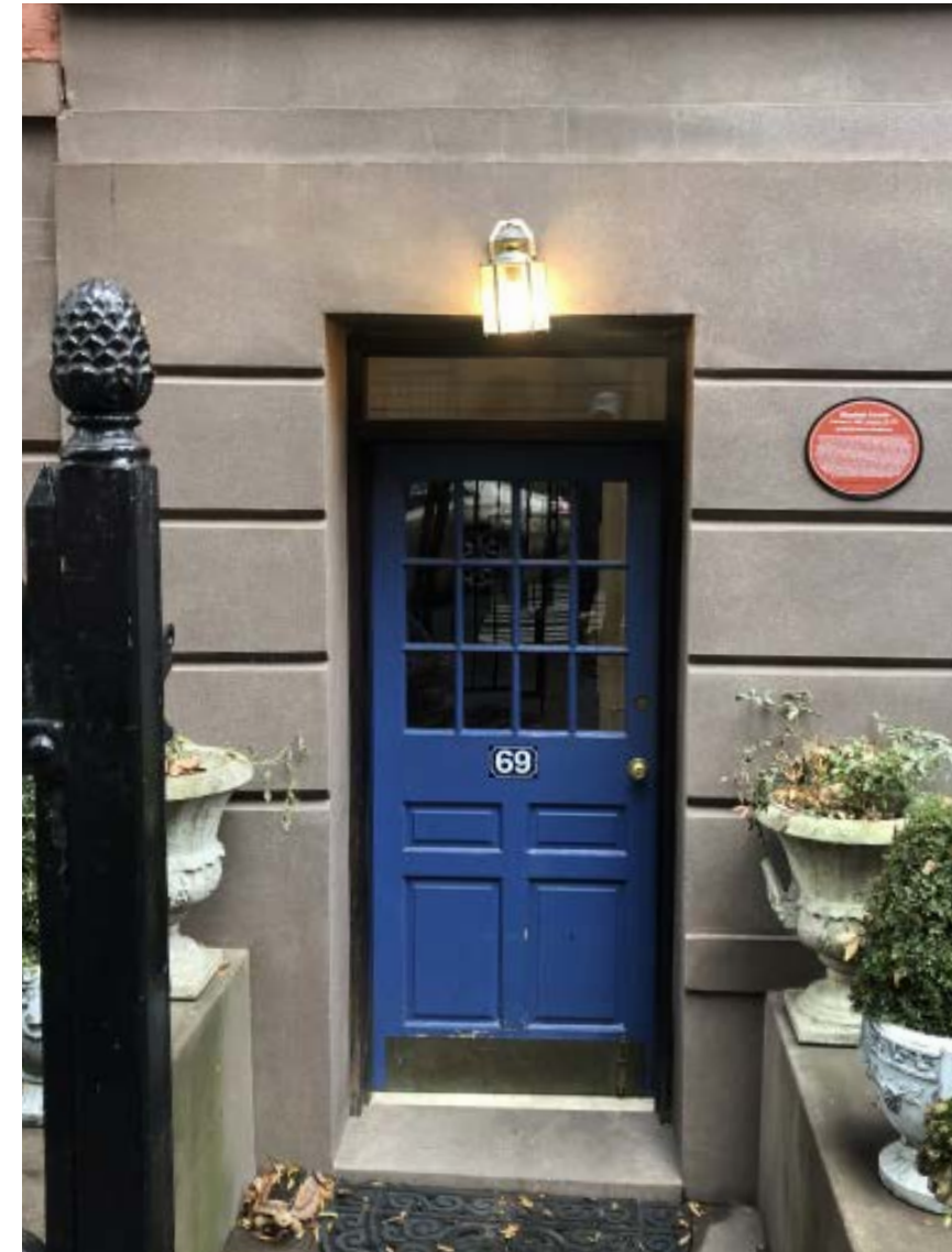
69 CHARLES STREET MAIN ENTRANCE
