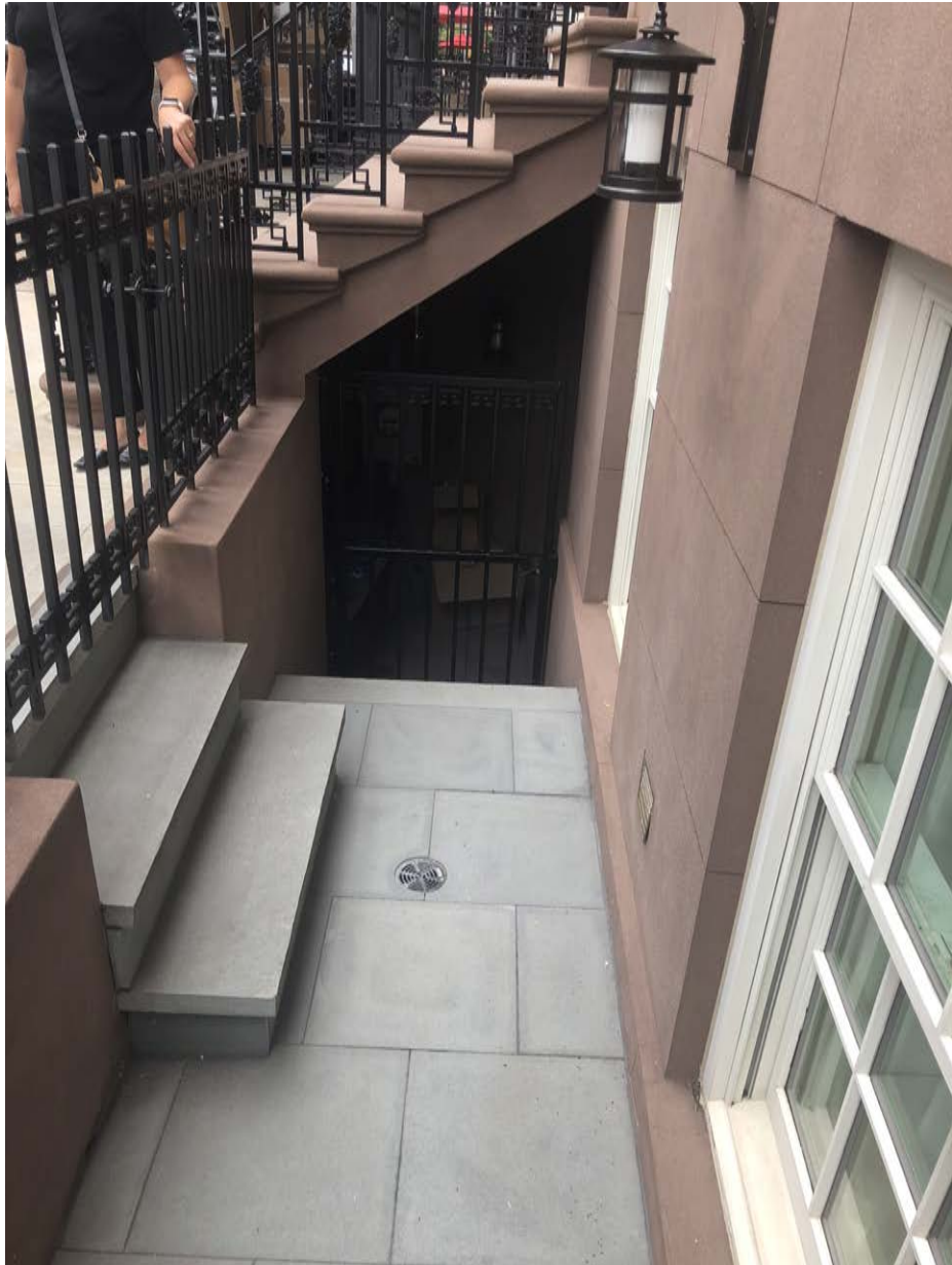
Existing areaway at 317
