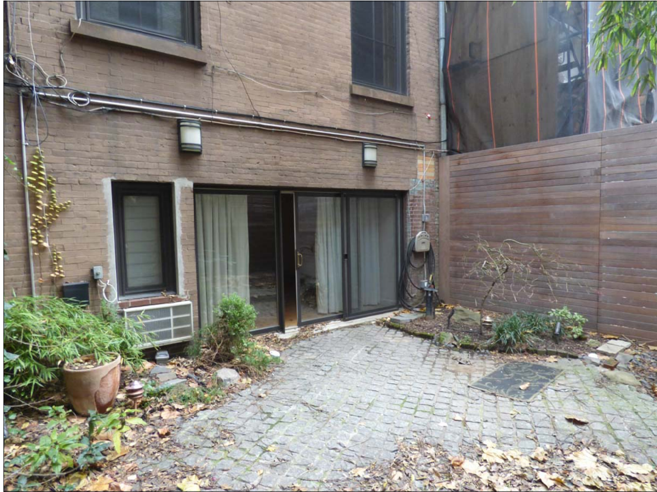
38 W10 Rear Elevation at Basement
