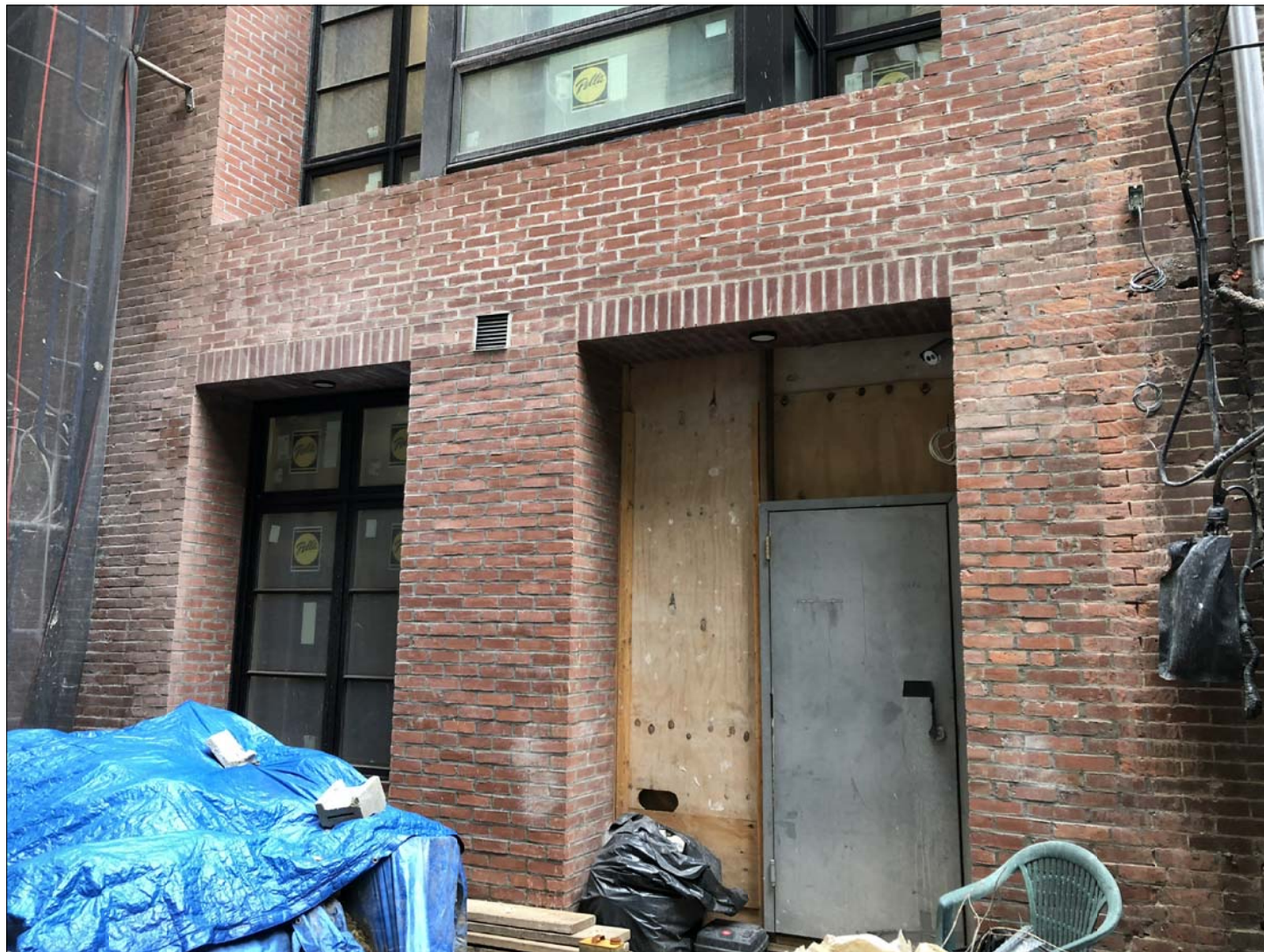
36 W10 Rear Elevation at Basement
