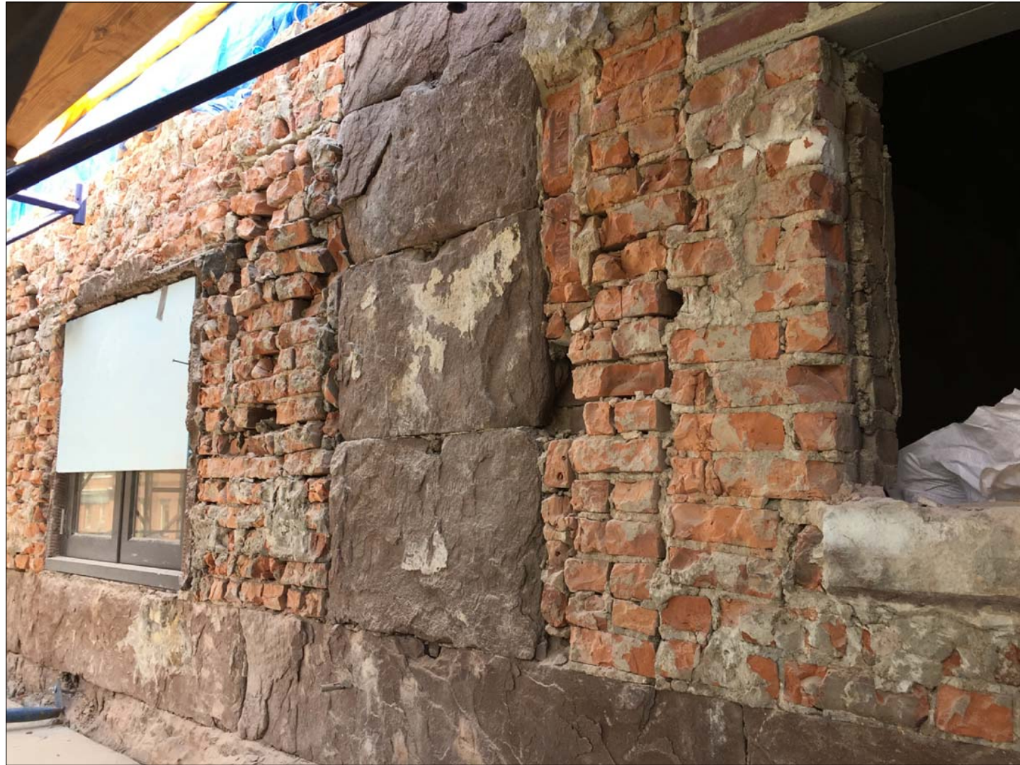
5TH FLOOR EXISTING BROWNSTONE BETWEEN NO. 36 & NO. 38
