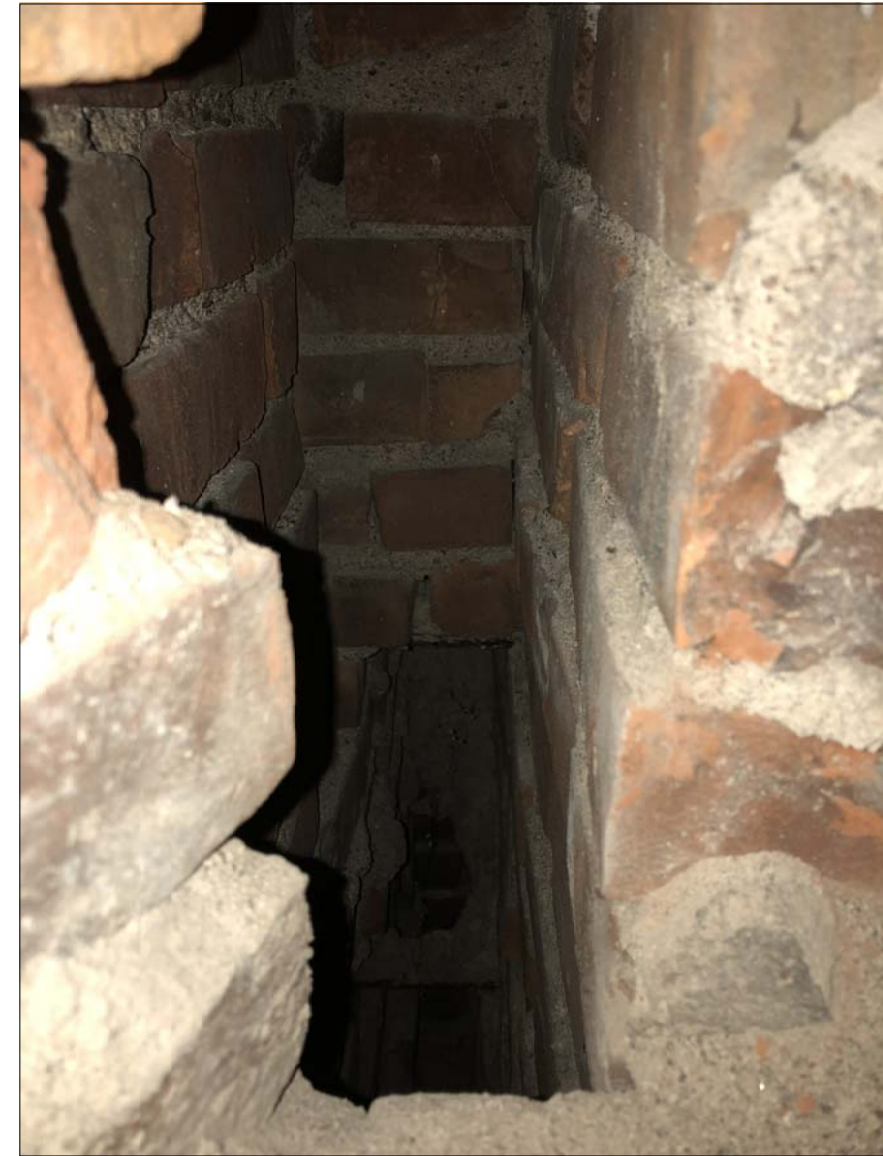
EXISTING FACADE CAVITY WALL AT 36 W10
