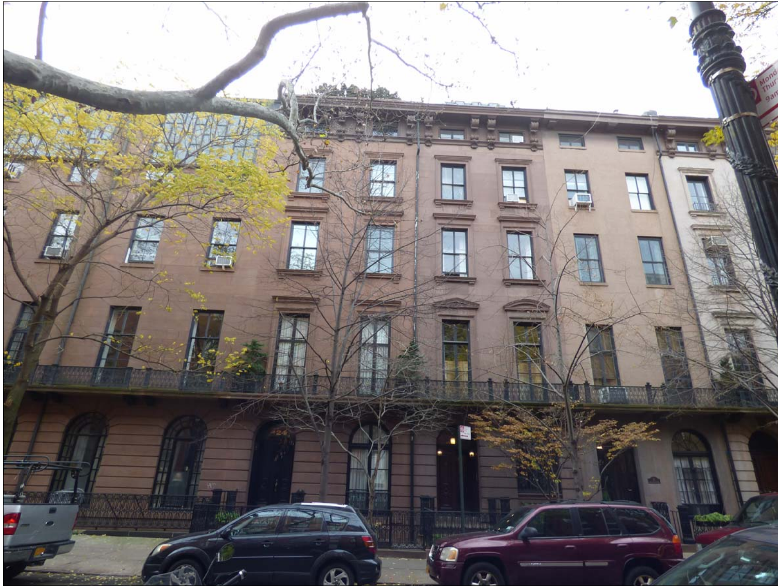
PHOTO OF 20, 22, 24, 26, 28, 30 W10 STREET FACADES
