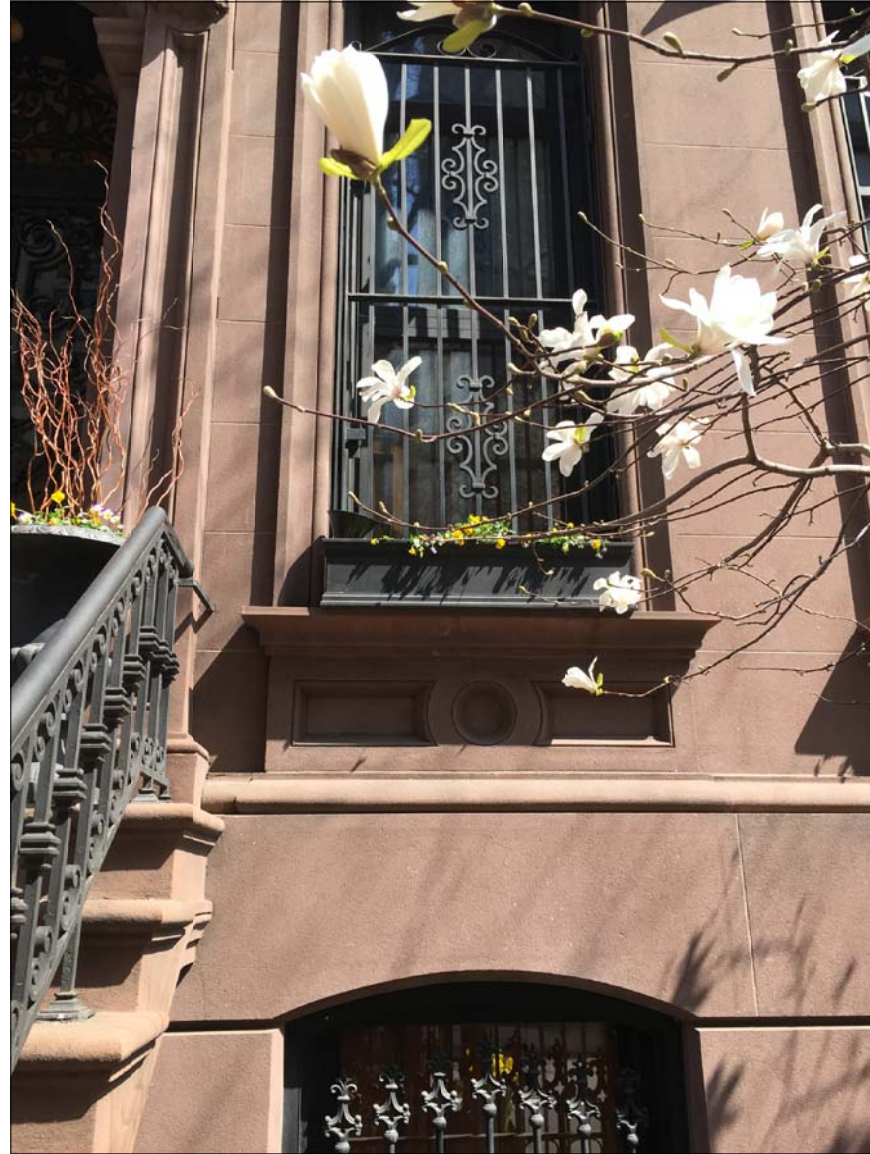
PHOTOS OF COMPLETED FACADE REPLACEMENT AT 129 EAST 35TH STREET UTILIZING CAST STONE
