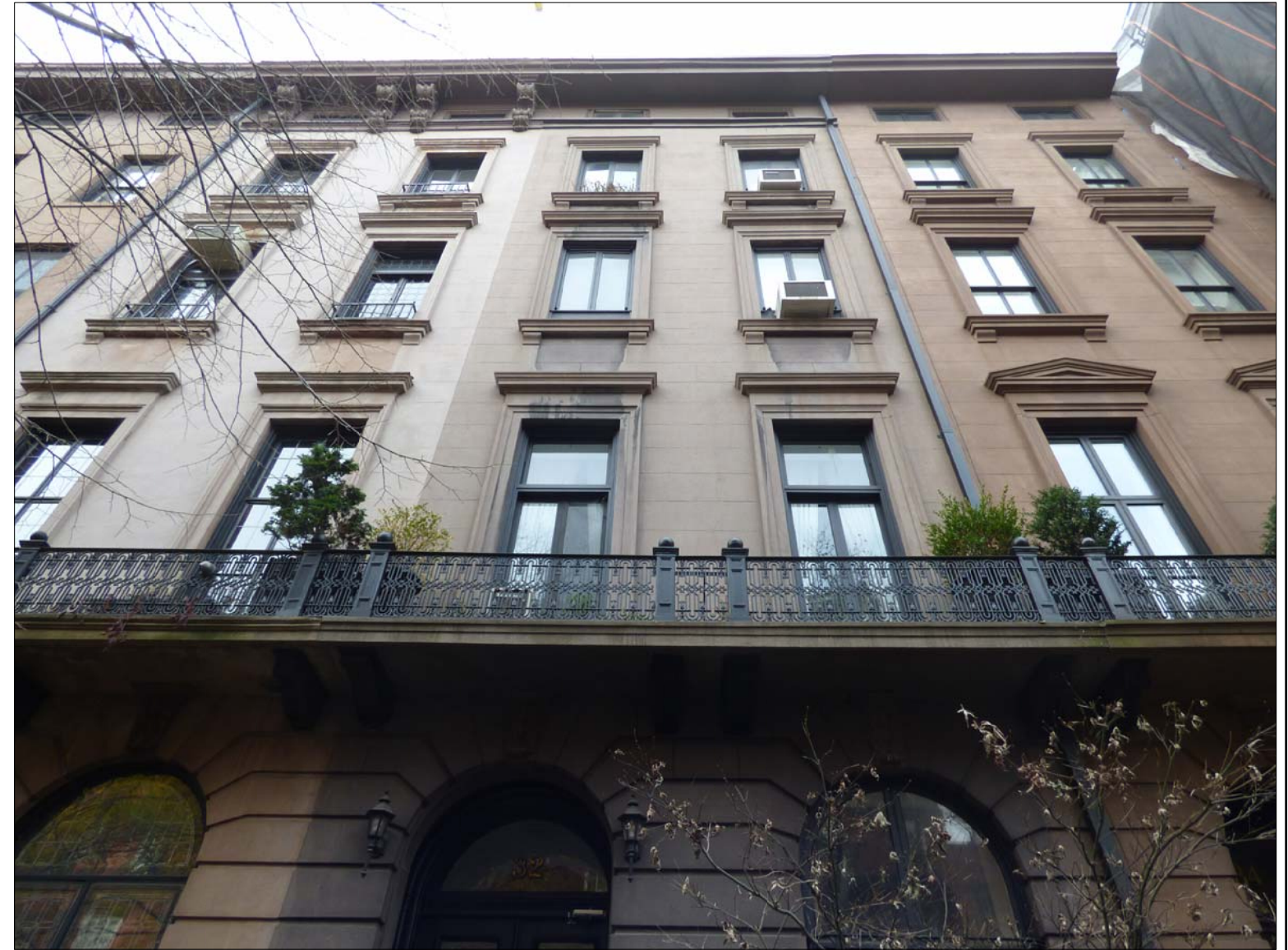
PHOTO OF 30, 32, 34 W10 STREET FACADES
