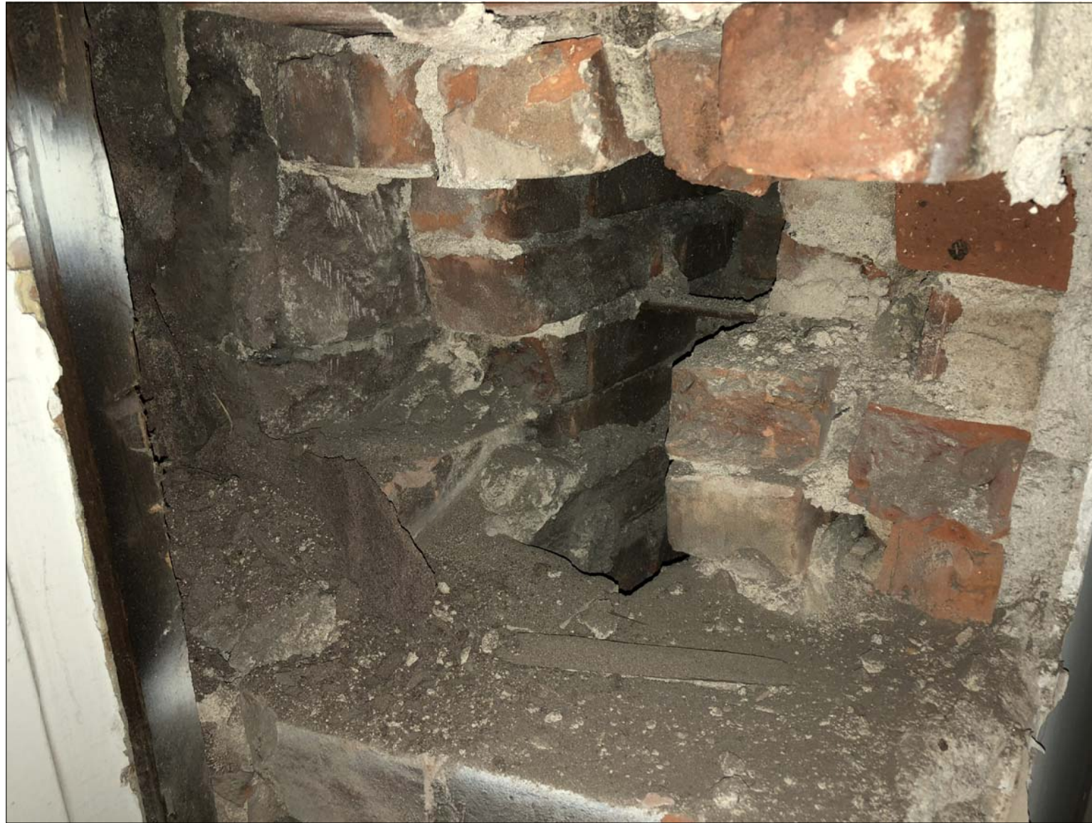
EXISTING FACADE CAVITY WALL AT 38 W10
