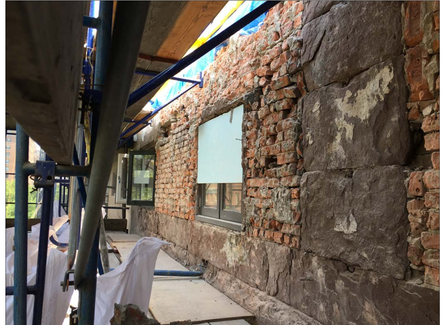
5TH FLOOR EXISTING BROWNSTONE BETWEEN NO. 36 & NO. 38
