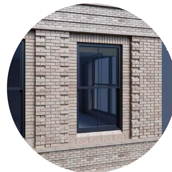
DETAIL 1: BRICK PIER & WINDOW SURROUND
