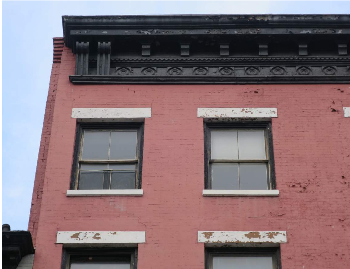
HISTORIC METAL CORNICE AND DETERIORATED WOOD WINDOWS
