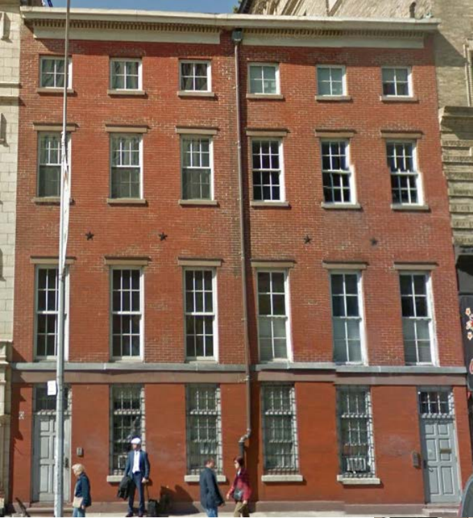
West side of 4 th Ave., btw. 11 th and 12 th Streets
