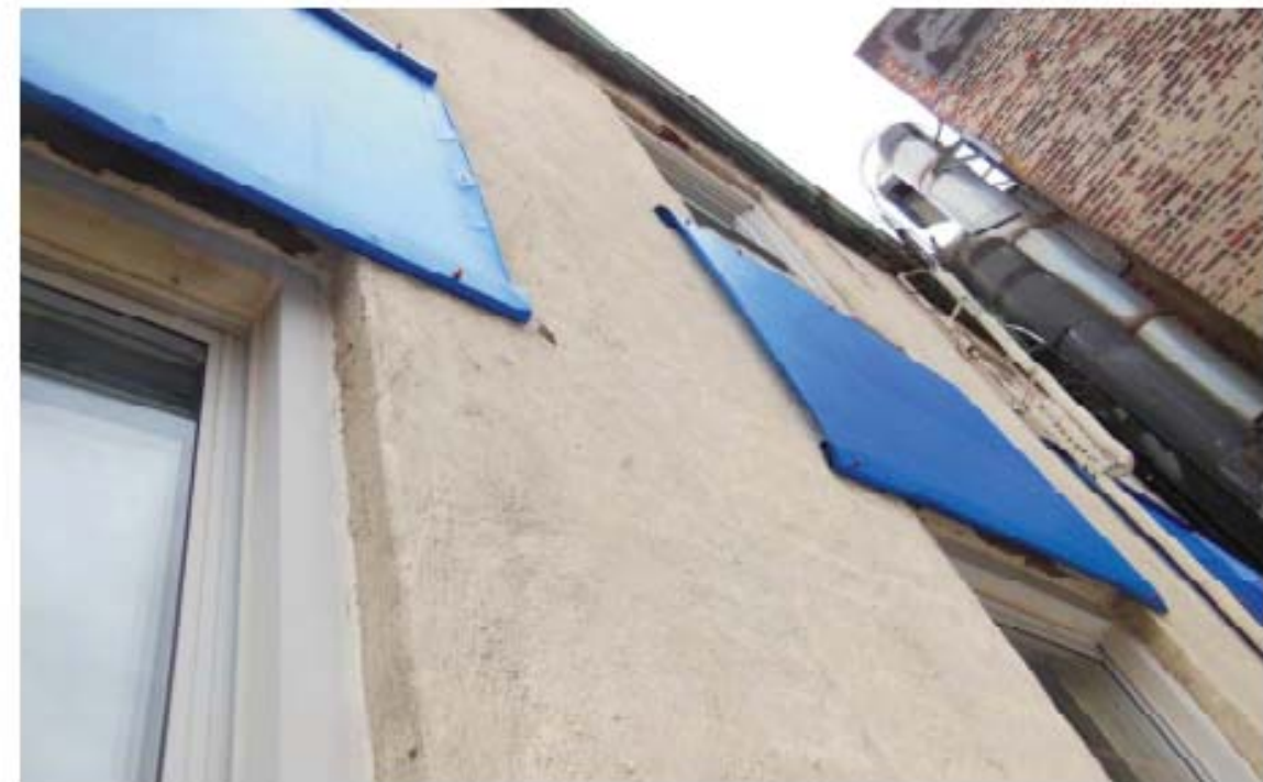
41 Greenwich-12 Rear facade
