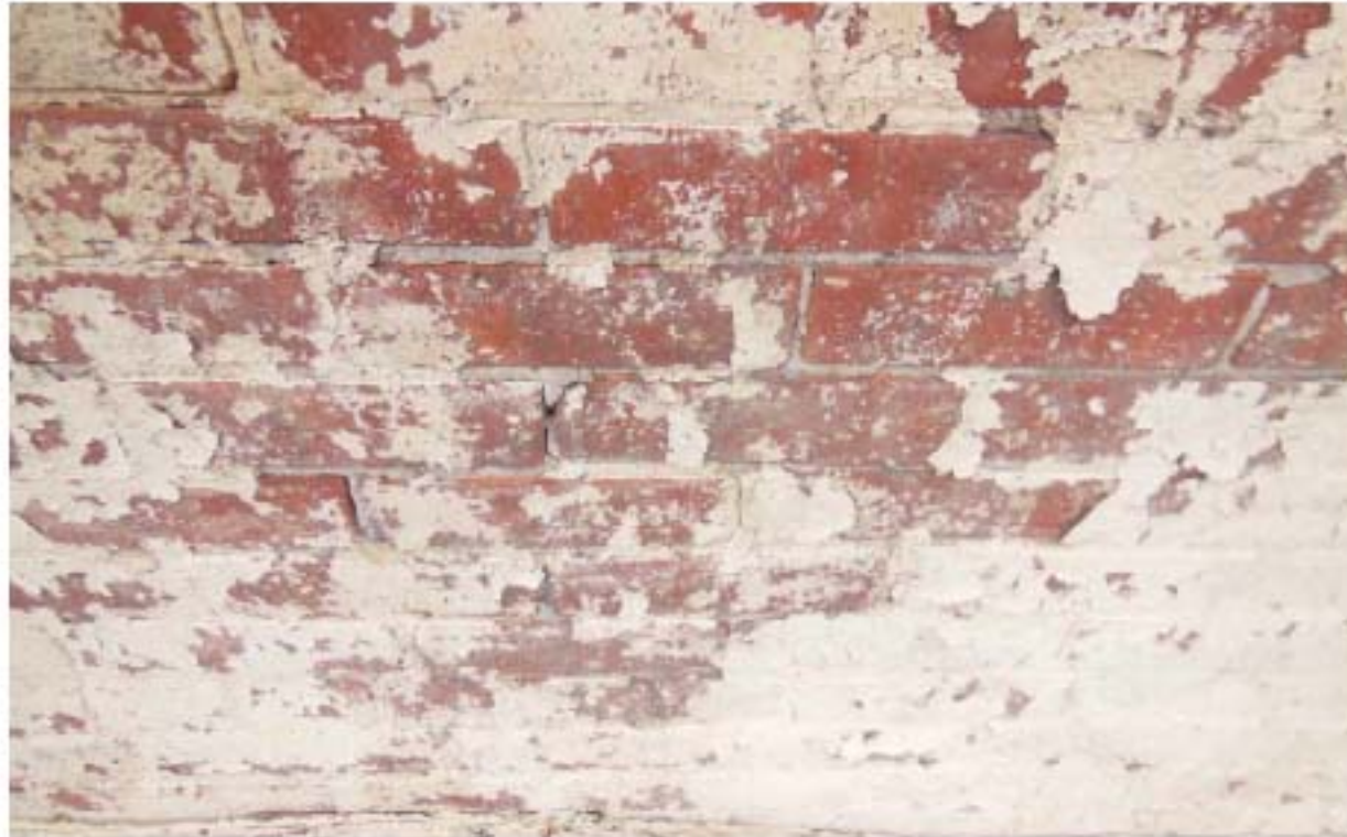
41 Greenwich-10 Rear facade
