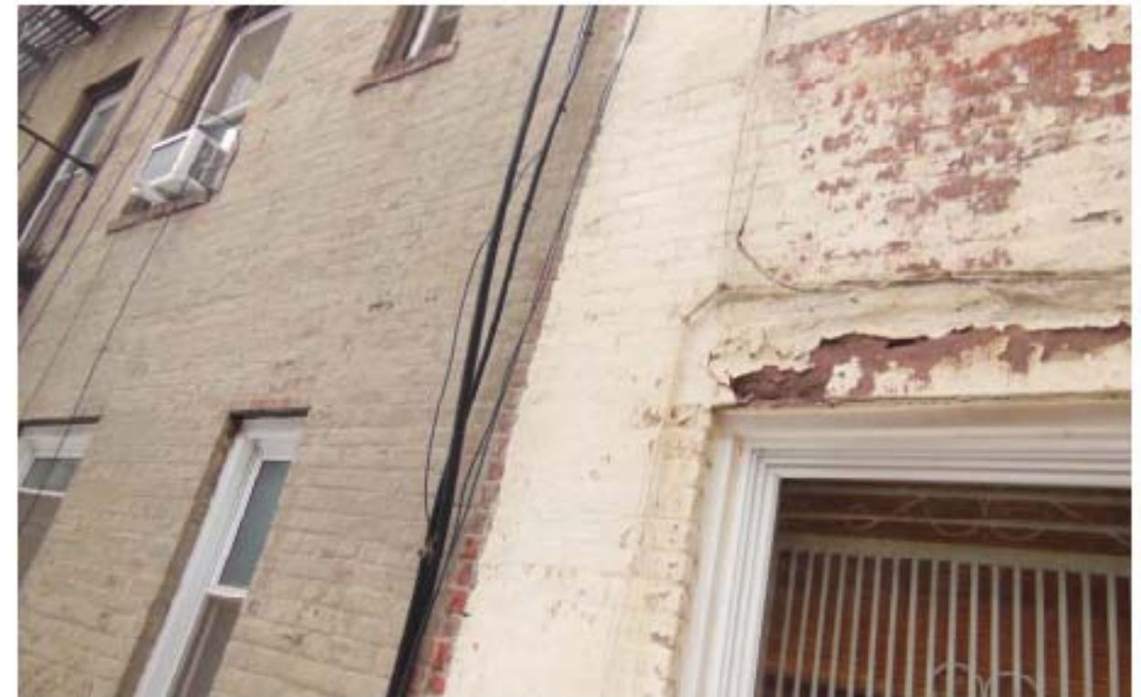
41 Greenwich-9 Rear facade
