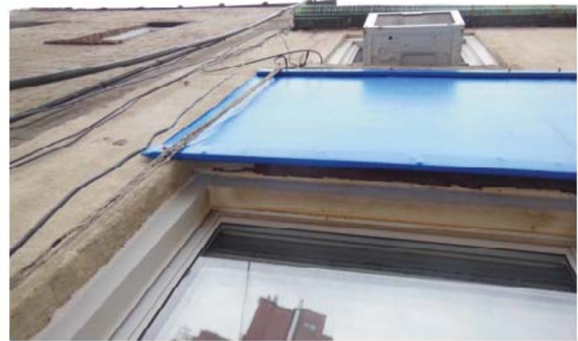
41 Greenwich-11 Rear facade
