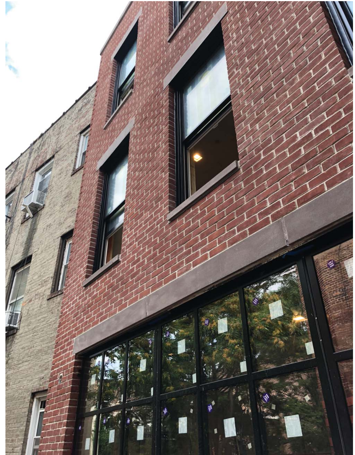
Rear Wall - Built Condition
