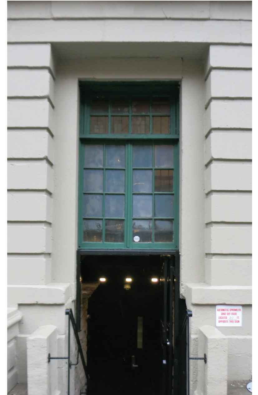
LPC Docket# 09-6497 Previously approved changes: - Removal of window & panel - New casement window
