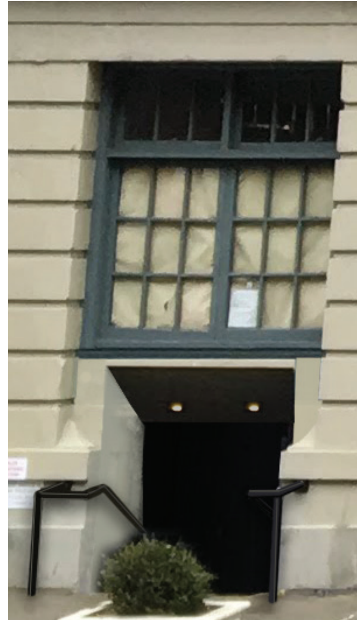
- Updated stair entryway - Historic style of window sill
