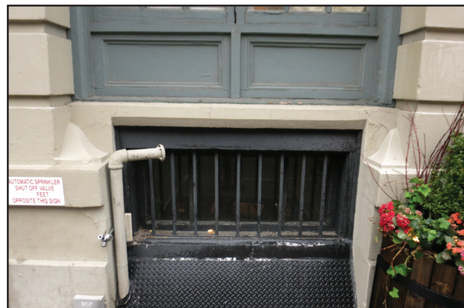
Existing - Basement Window With Grill
