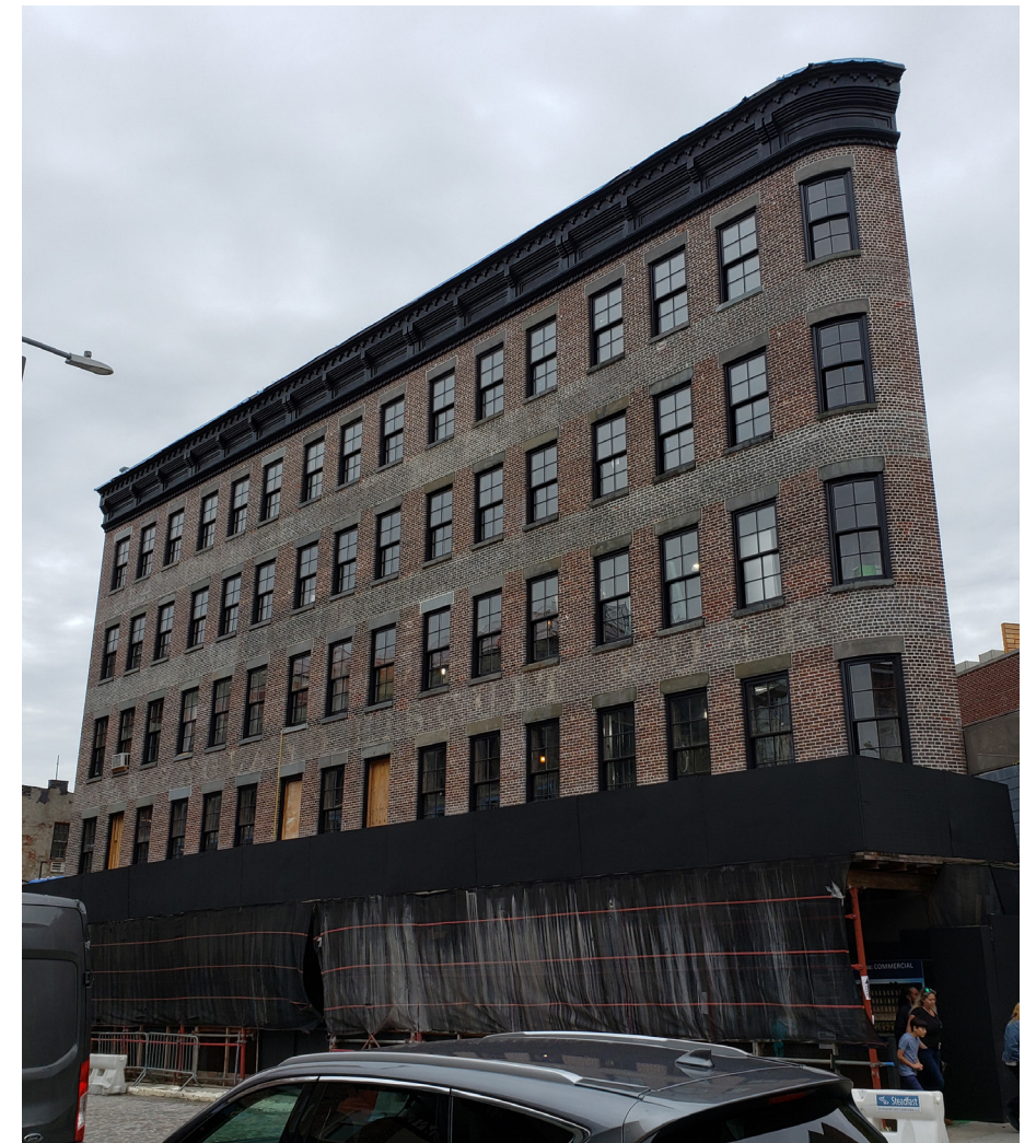
October 2019: Current condition, undergoing renovation
