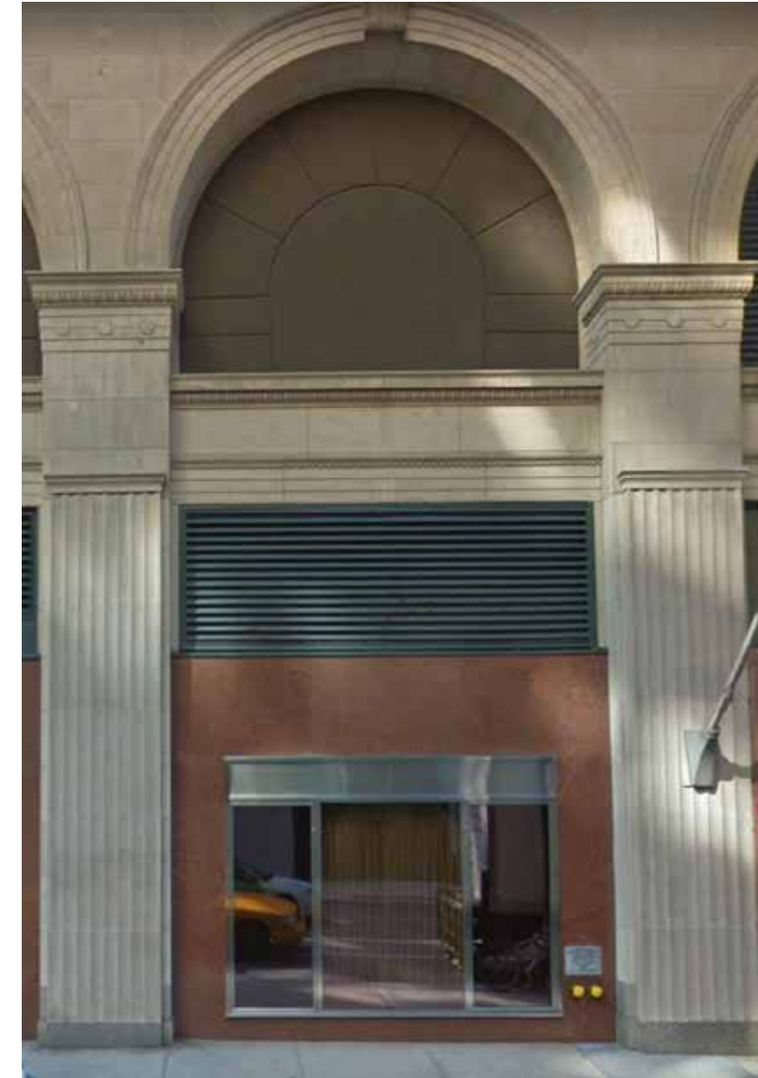
3 | 2014 Bay Condition - Bay 12
