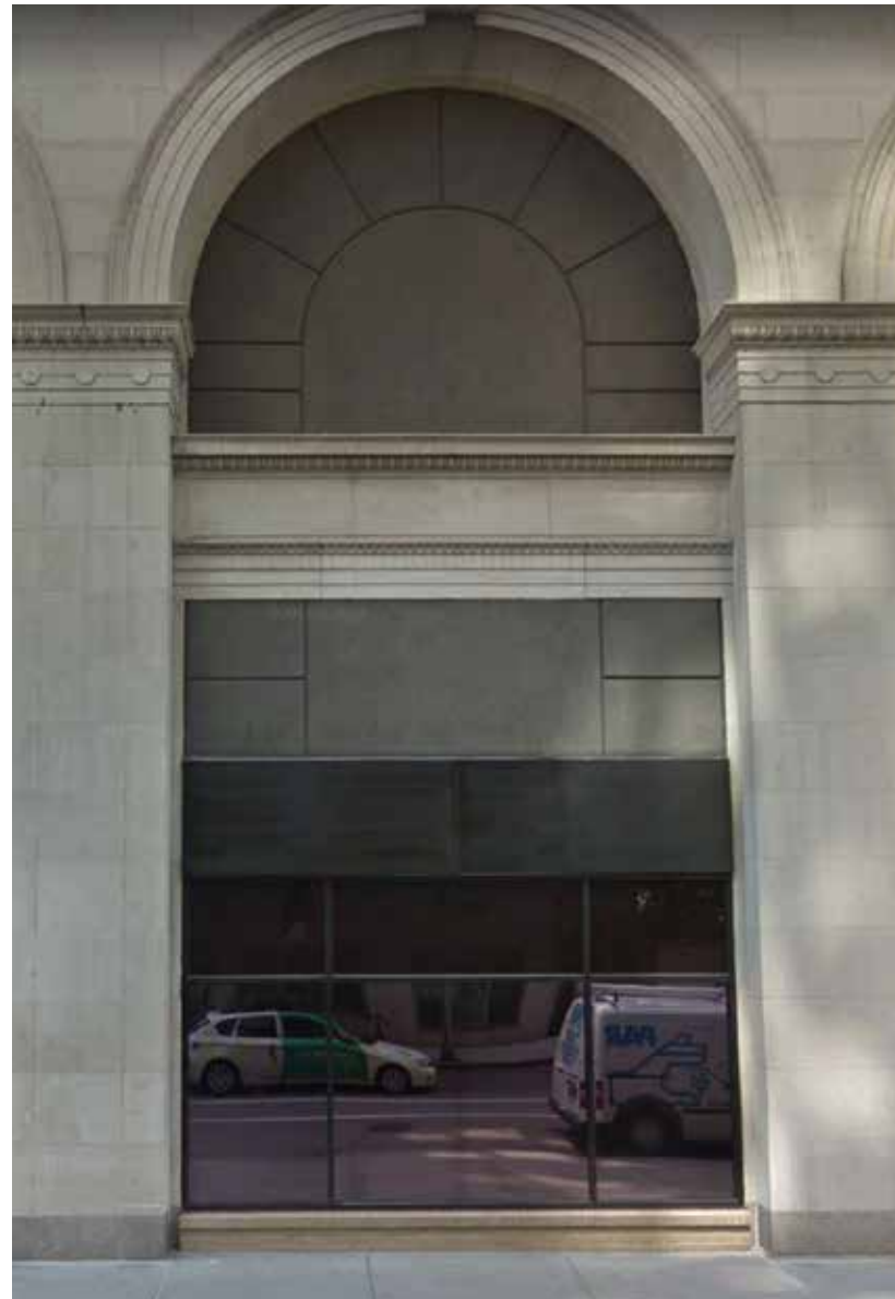
1 | 2014 Bay Condition - Bay 10
