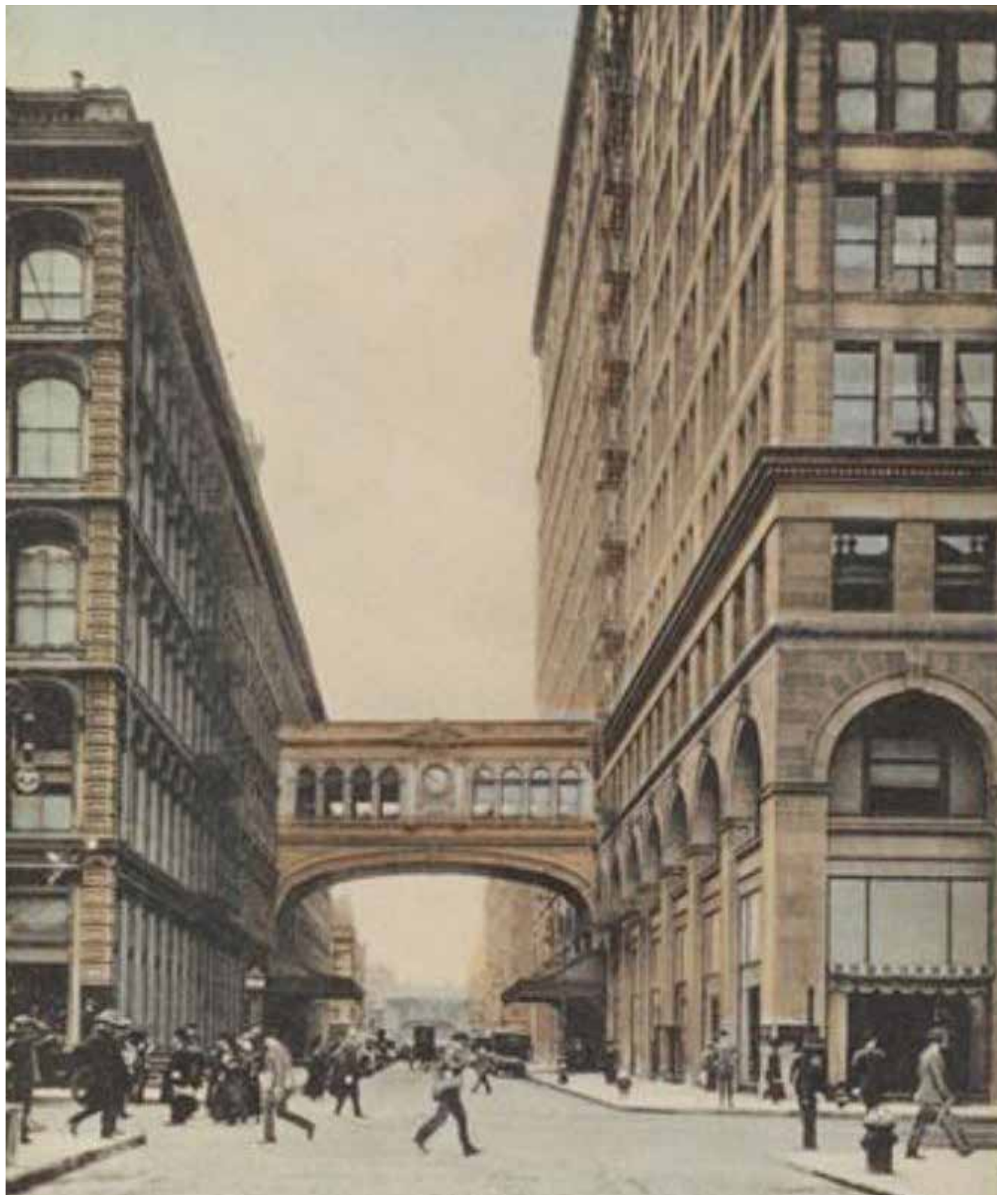
1 | Bridge of Progress (1924)
