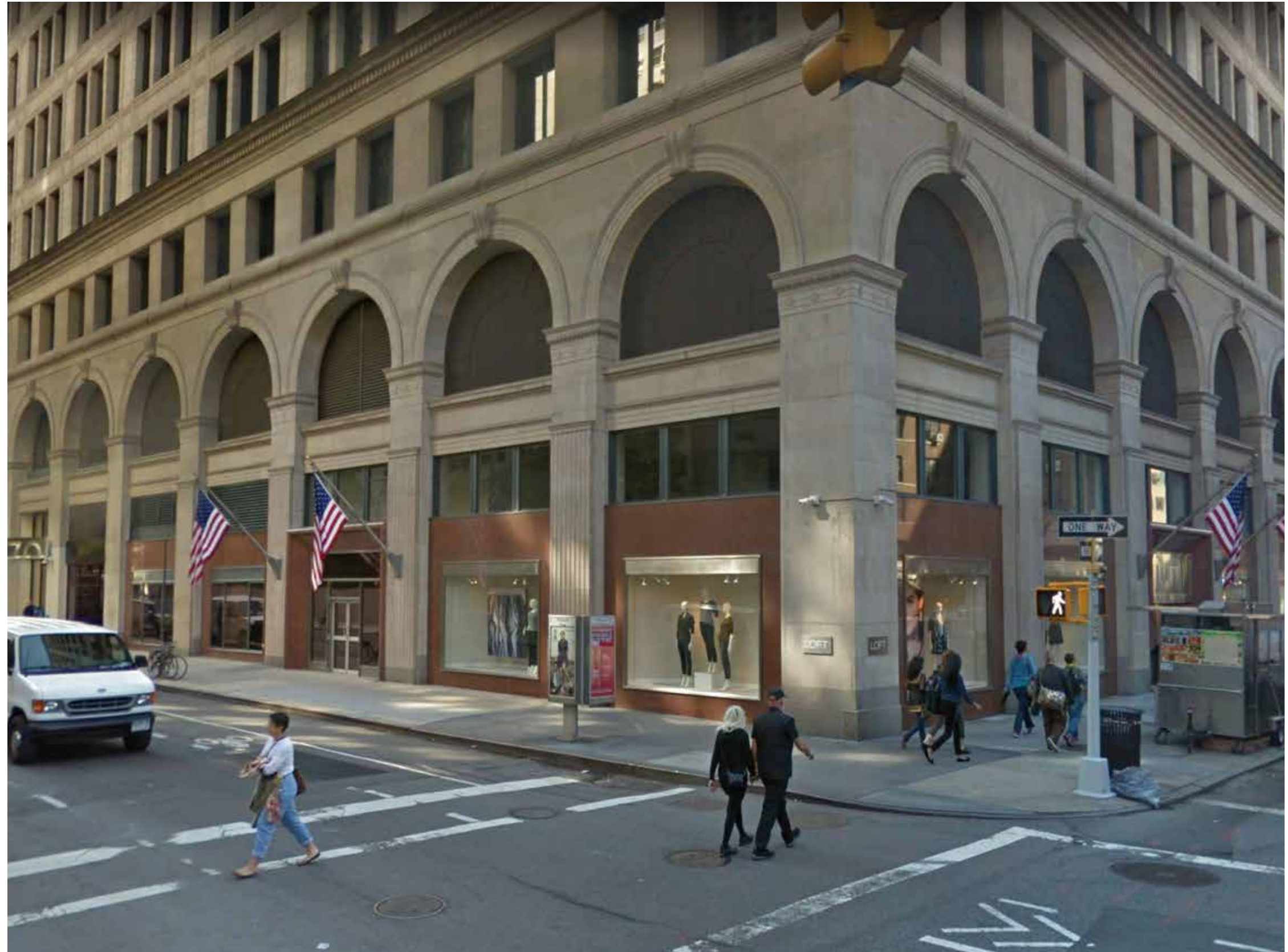
1 | Overall View of NW Corner Current Config. (2014)
