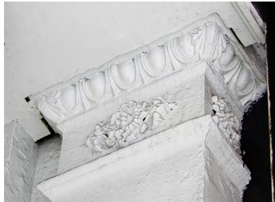
ORIGINAL CAST IRON SIDE PILASTER
