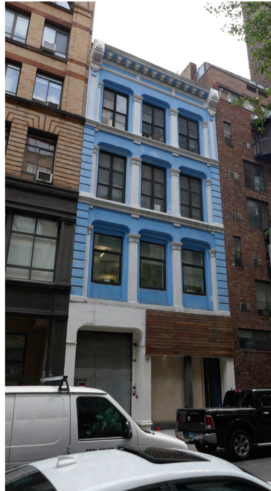
EAST 12TH STREET FACADE & STOREFRONT
