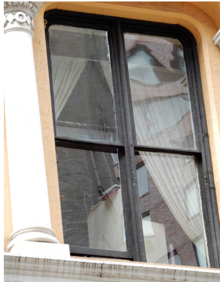
EARLY OR ORIGINAL PAIRED 1/1 SASH
