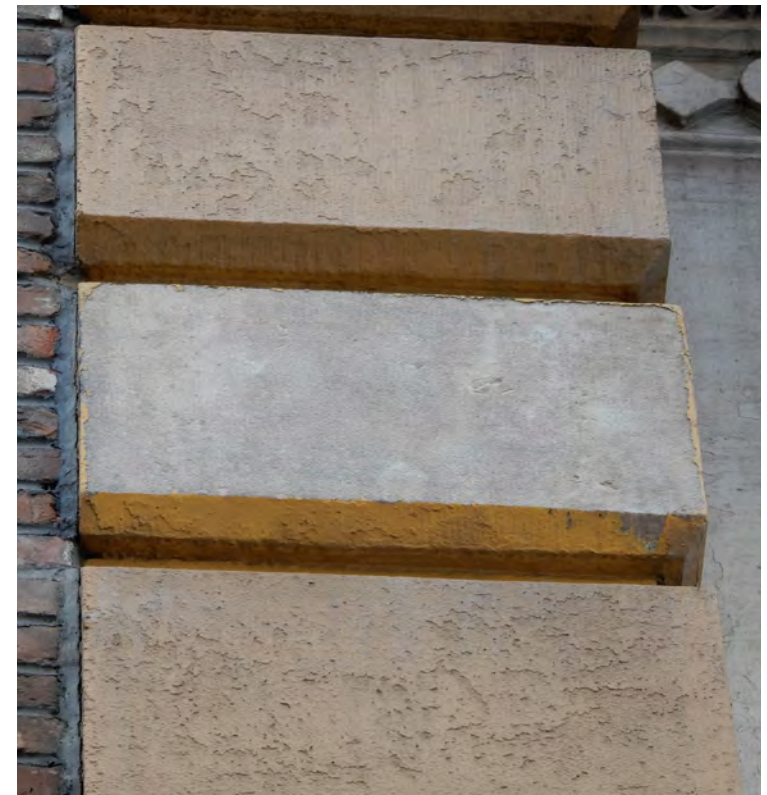
QUOIN AFTER TEST CLEANING
