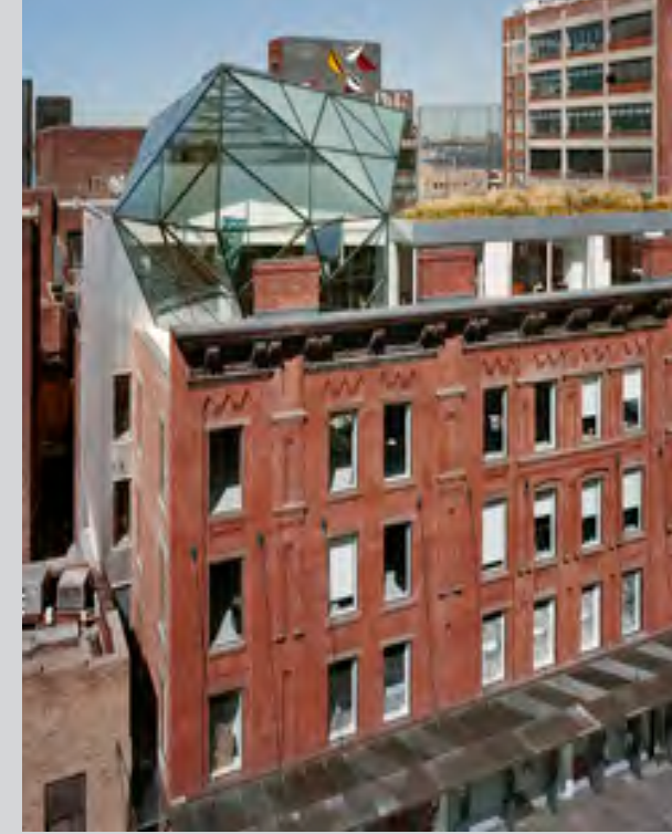
DVF STUDIO HEADQUARTERS - WORK AC
