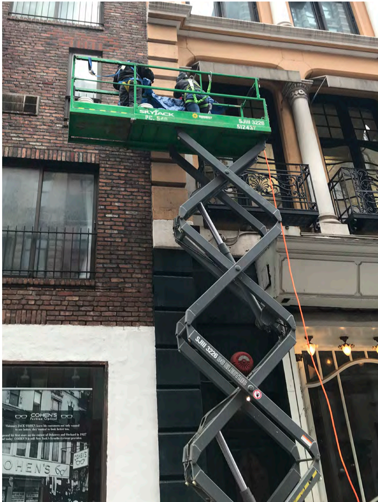
SECOND FLOOR QUOIN USED FOR MICRO ABRASIVE TESTING WITH; 1. CALCIUM CARBONATE Z5 GRAIN SIZE 2. GARNET, 120 MESH 3. CRUSHED WALNUT SHELLS, 35/60 MESH
