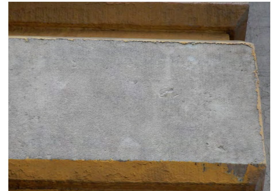
QUOIN AFTER ABRASIVE CLEANING WITH CRUSHED WALNUT SHELLS AT 40PSI
