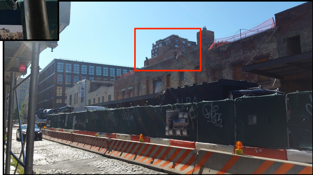
838 Greenwich lot line wall viewed from the west, mid-block on Gansevoort.
