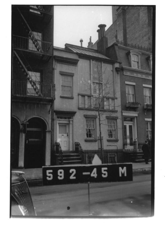
Tax photo circa 1940 showing roof leaders attached to cornice molding. Note extension of façade wall to form parapet on either side of the studio windows.
