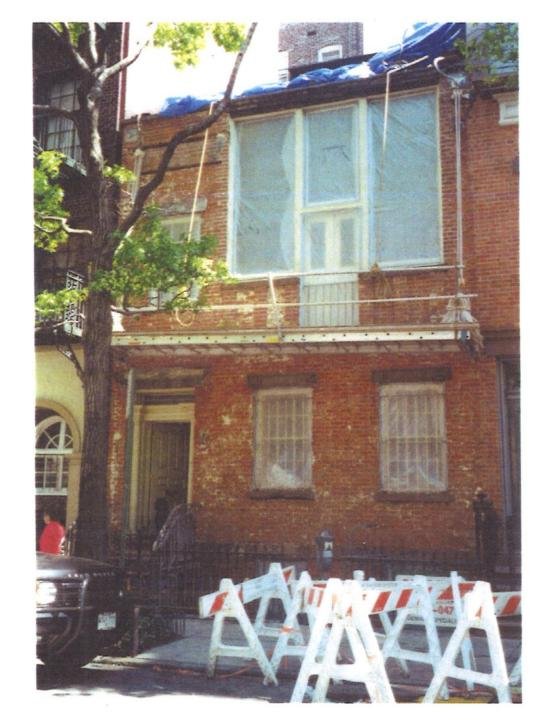
Façade during Adami restoration showing brick after cleaning and before repointing. Windows not yet replaced in this picture. Taken in 1997.
