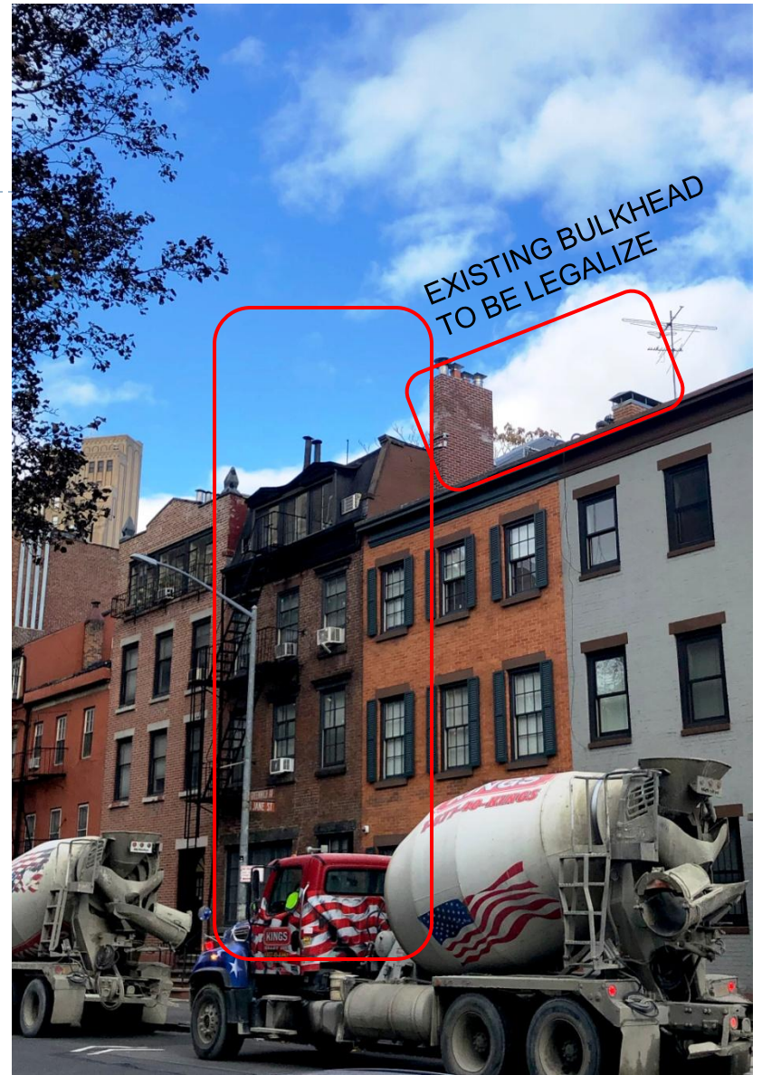
EXPOSURE OF BUILDING LOOKING NORTH BOUND ON GREENWICH AVENUE
