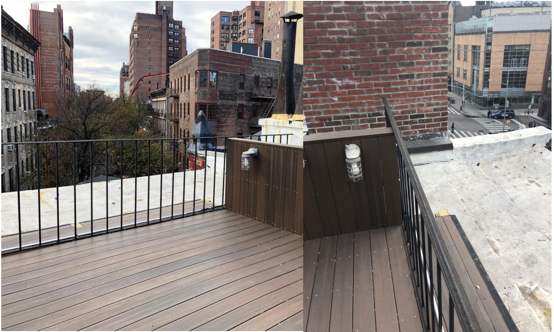
Bulkhead(s) On The Southern Side
