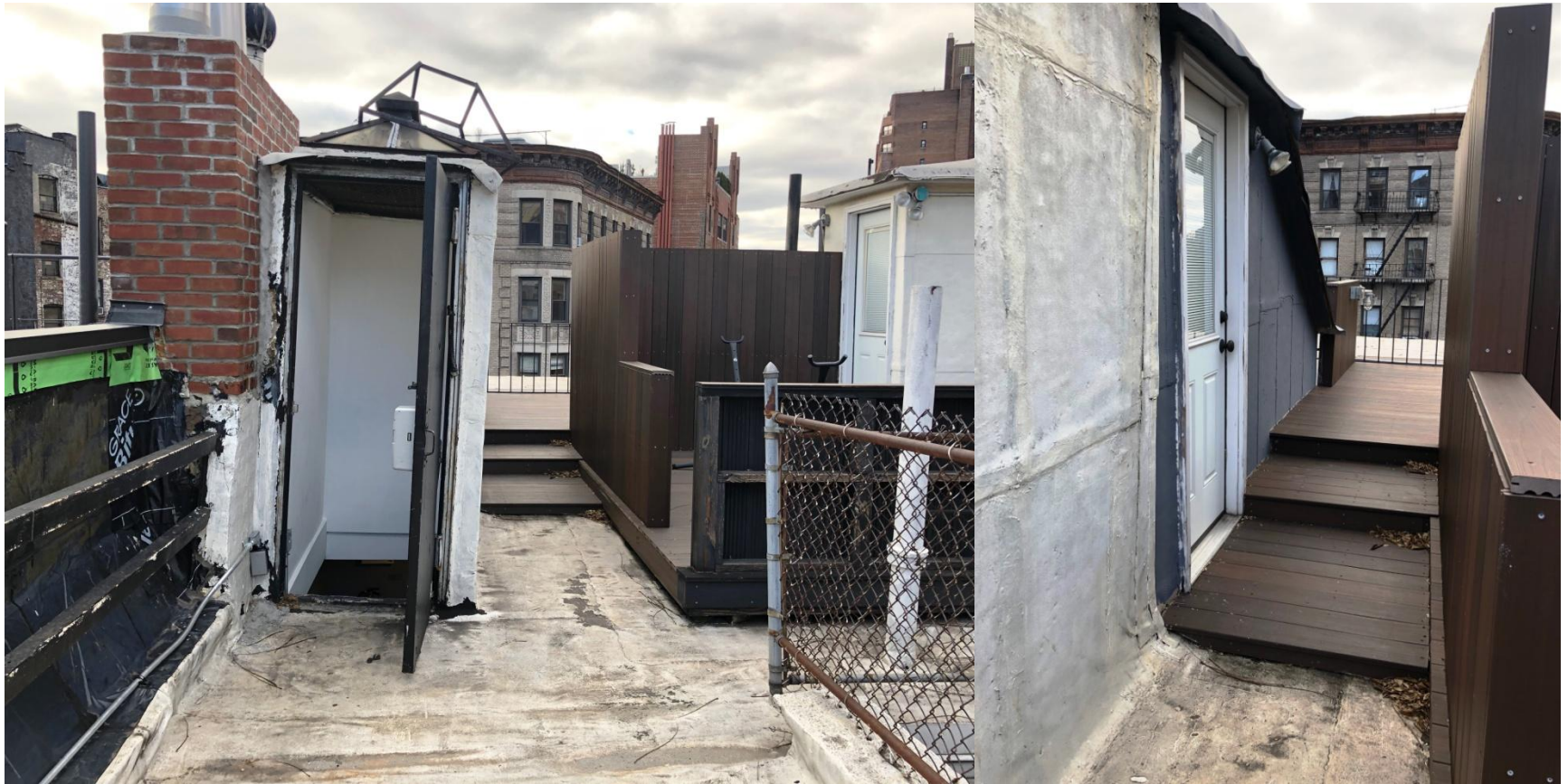
Bulkhead(s) On The Southern Side
