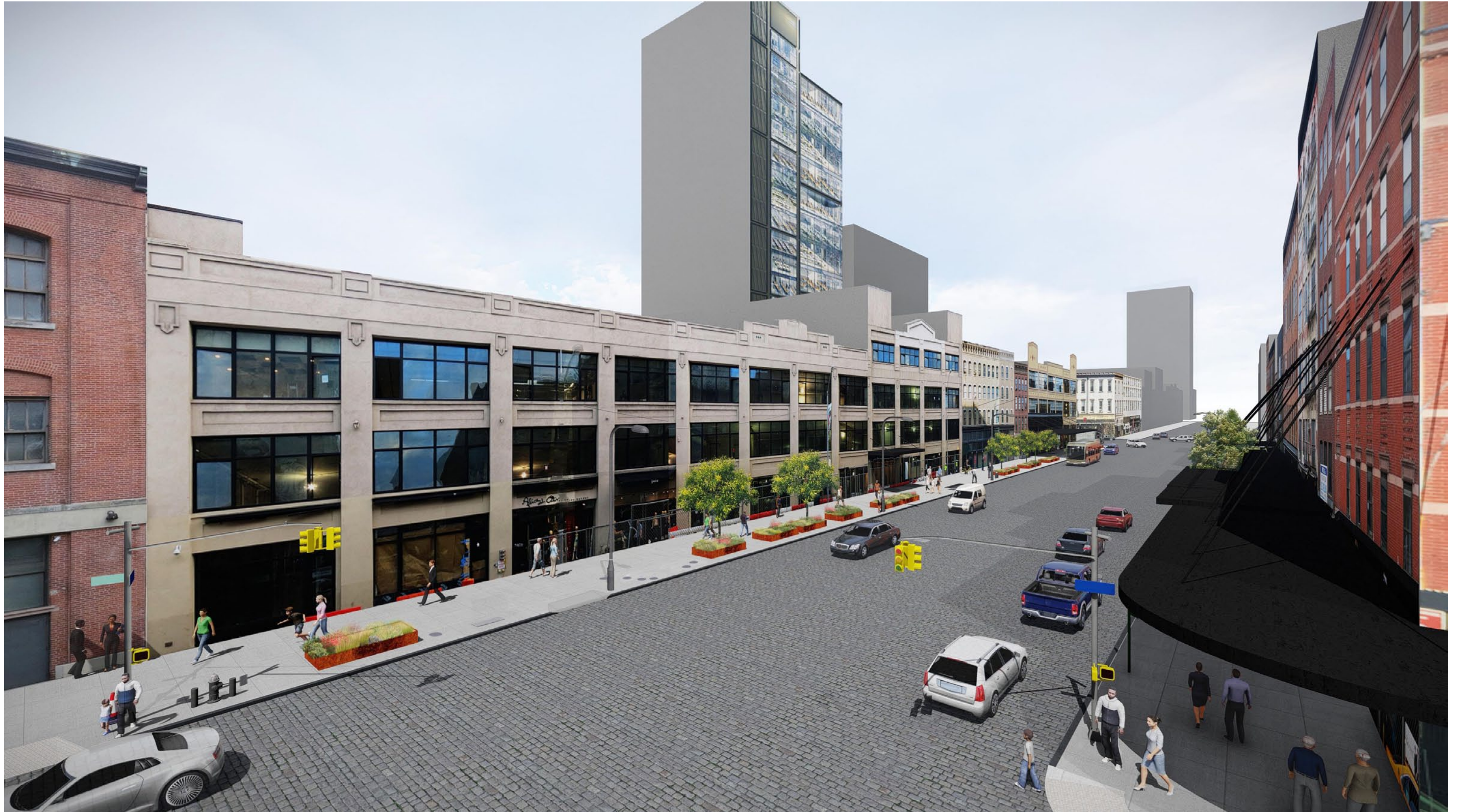
This view shows the proposed planters with “Highline” type herbaceous planting and sporadic street trees North side of 14th Street, looking northeast
