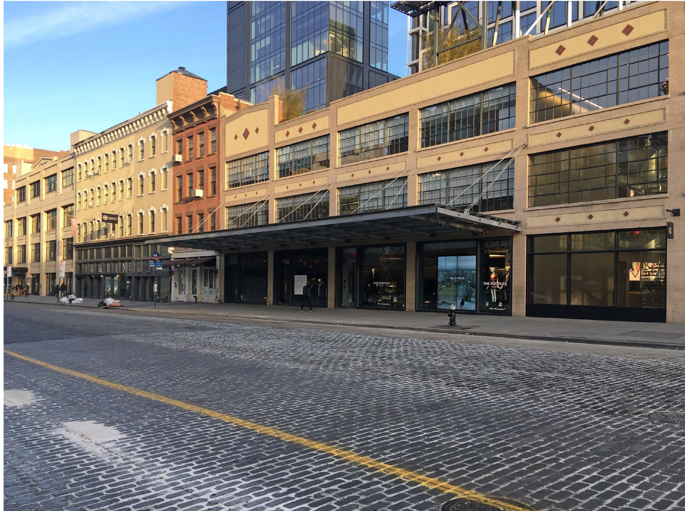
Existing view North side of 14th Street
