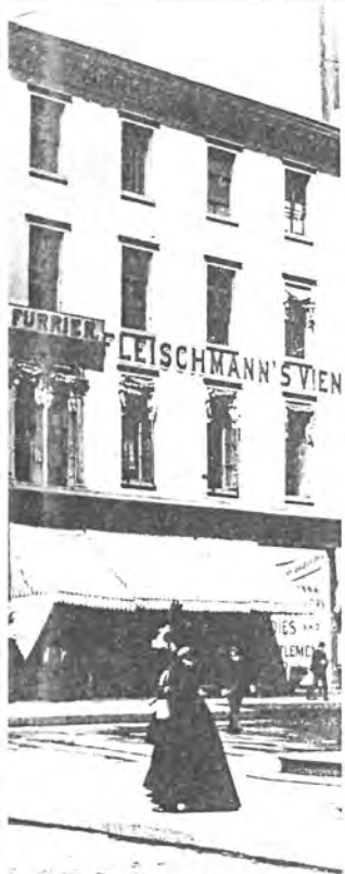
of Broadway and 10th Street, ed between Grace Church and which produced its own baked along Ladies' Mile. (The Byron
