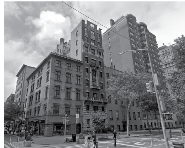
14-16 FIFTH AVENUE IS THE FIVE-STORY BUILDING IN THE CENTER. A DEVELOPER WANTS TO REPLACE IT WITH A 244 FT. TALL TOWER
