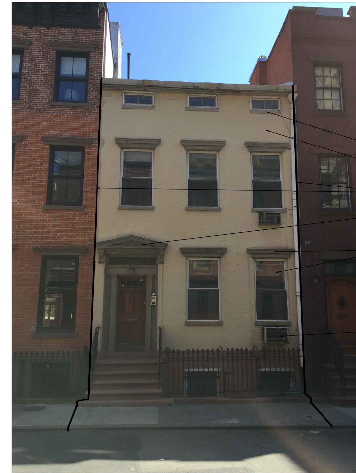
3 EXISTING NORTH FACADE BUILDING PHOTO Scale: NTS
