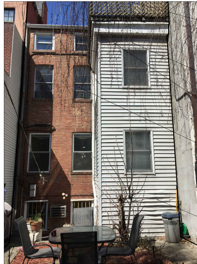
2 EXISTING SOUTH FACADE BUILDING PHOTO Scale: NTS
