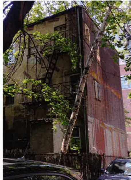
metal panel, view from rear
