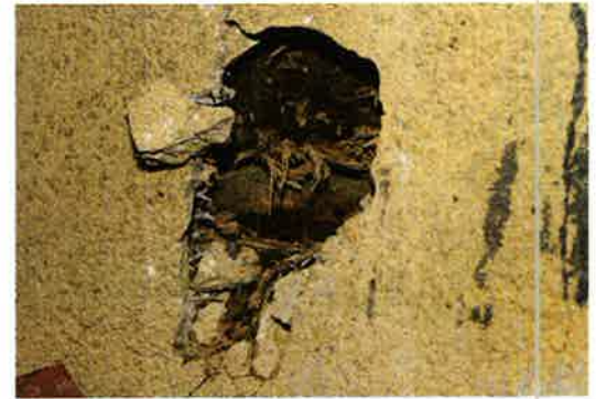
probe at rear facade showing evidence of clapboard siding under stucco
