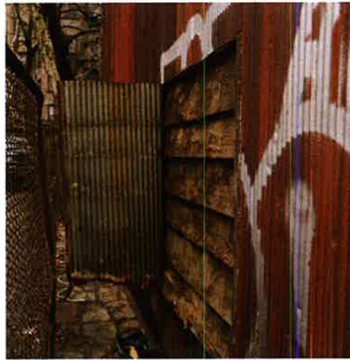
view of clapboard siding under metal panel
