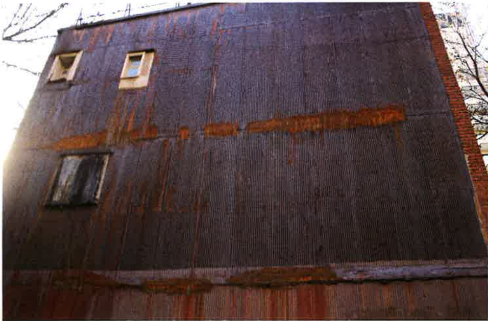
metal panel, view from neighboring lot
