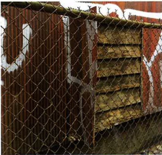
view of clapboard siding under metal panel
