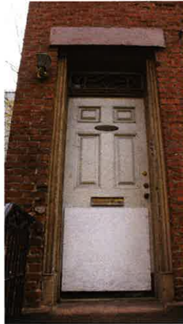
Existing entry door
