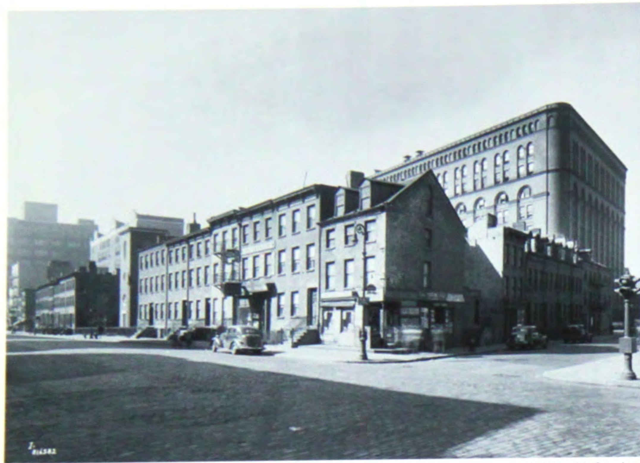
Archives Building, 11 Stories
