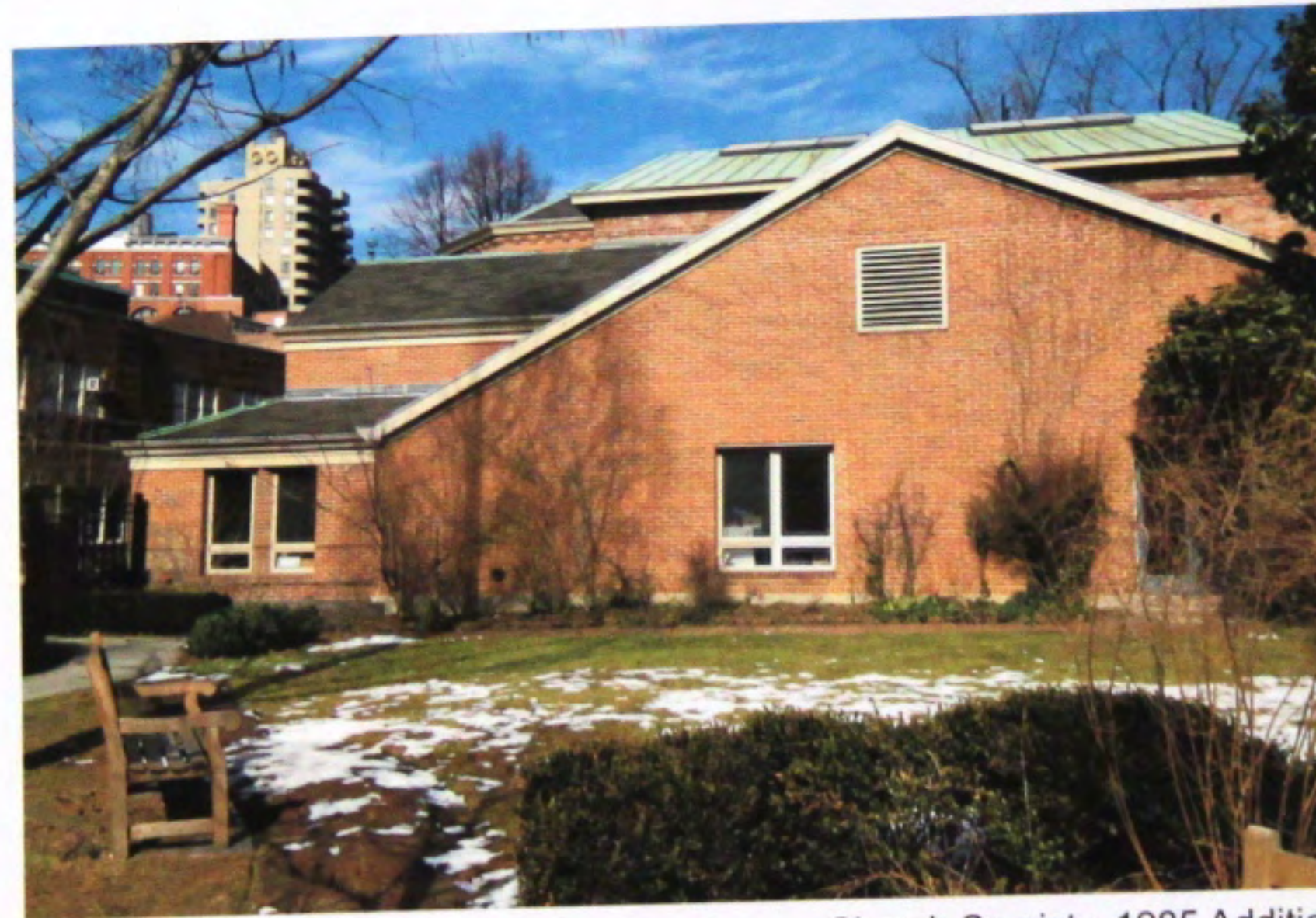
Church Sacristy, 1985 Addition
