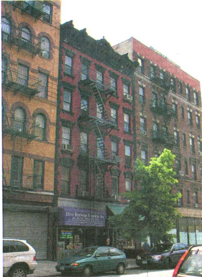
Built in 1873, 52 Carmine Street is a characteristic pre-Law tenement. It was originally built with no air shafts or side windows, although it was given elaborate cornices that remain intact.
