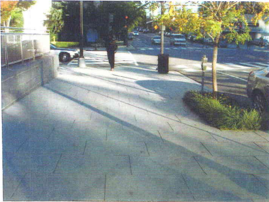
NYC DOT Standard Tinted Concrete
