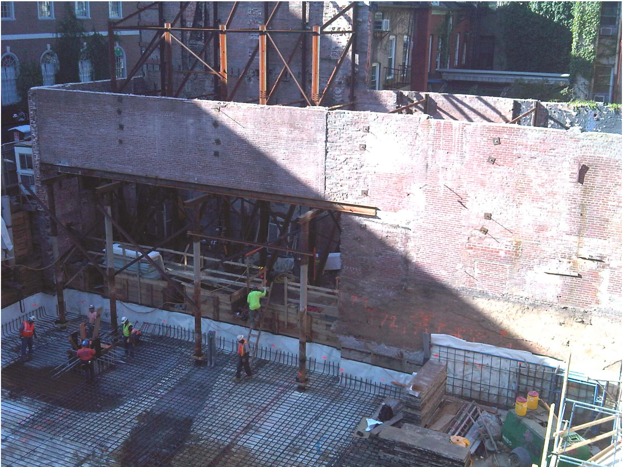
Demolition of Provincetown Playhouse & Apartments - 09/01/2009
