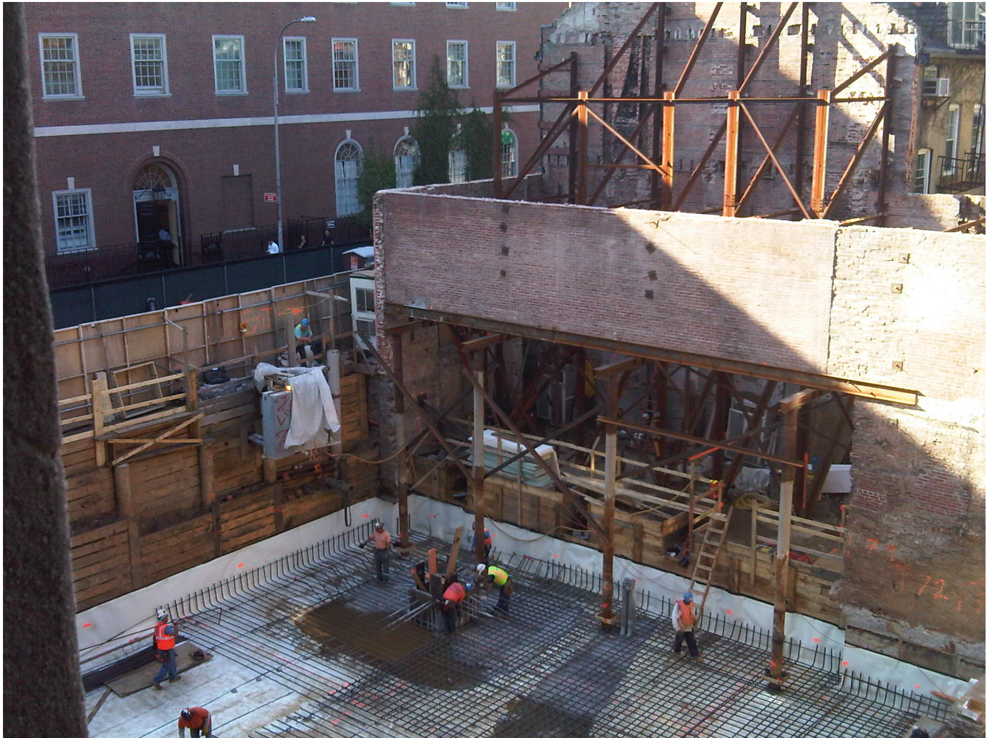
Demolition of Provincetown Playhouse & Apartments - 09/01/2009
