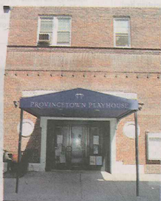
ANDREA MOHIN/THE NEW YORK TIMES 133-139 MACDOUGALL STREET N.Y.U. is renovating this longtime theater.
