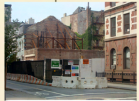
NYU begins demolition of Provincetown Playhouse and Apartments without landmark status
