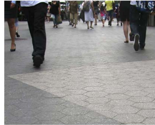
EXAMPLE OF HEX. ASPHALT PAVER AT UNION SQUARE
