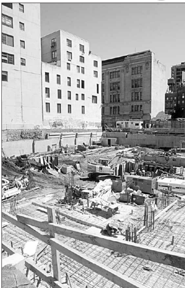
Construction has already started at 246 Spring St. in SoHo. (Jefferson Siegel)
