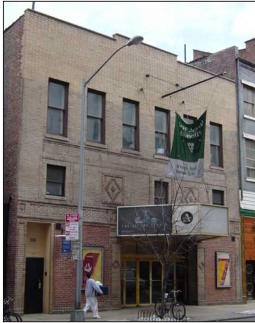
The Former Circle in the Square Theater at 159 Bleecker Street, before demolition began
